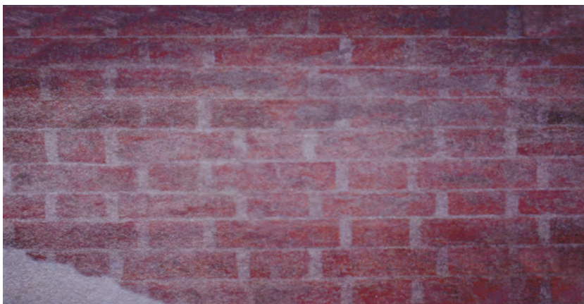
Fig. 1 - Venice, Santo Stefano Church: decoration reproducing a dummy brickwork, called as regalzier , on the right side of the building; XV th century.
