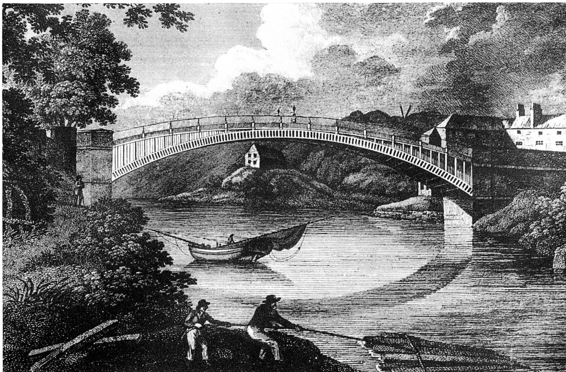
Fig. 5 The cast-iron bridge at Yarm, designed by Thomas Wilson; it collapsed in 1806 before being opened to traffic. [J. Graves, The History and Antiquities of Cleveland (Carlisle, 1808)]
