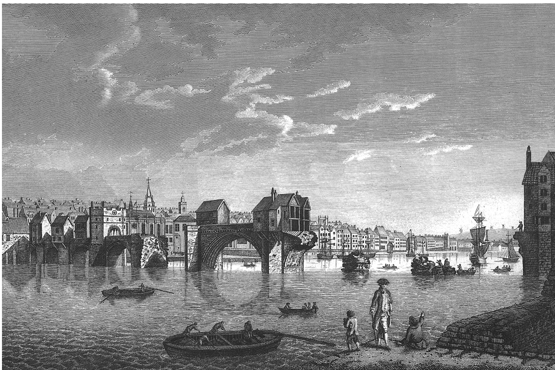
Fig. 2 The ruins of Newcastle bridge following the flood of 16/17 November 1771. [J. Brand, The History and Antiquities . . . of Newcastle (London, 1789)]
