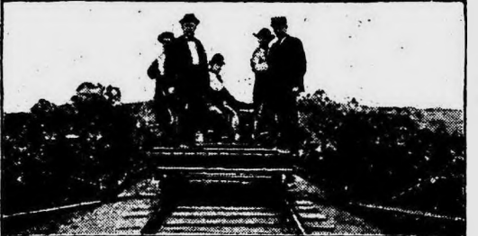
Cutting Weeds on a Railroad With Gasoline Power Instead of Slow-Going Scythes.
