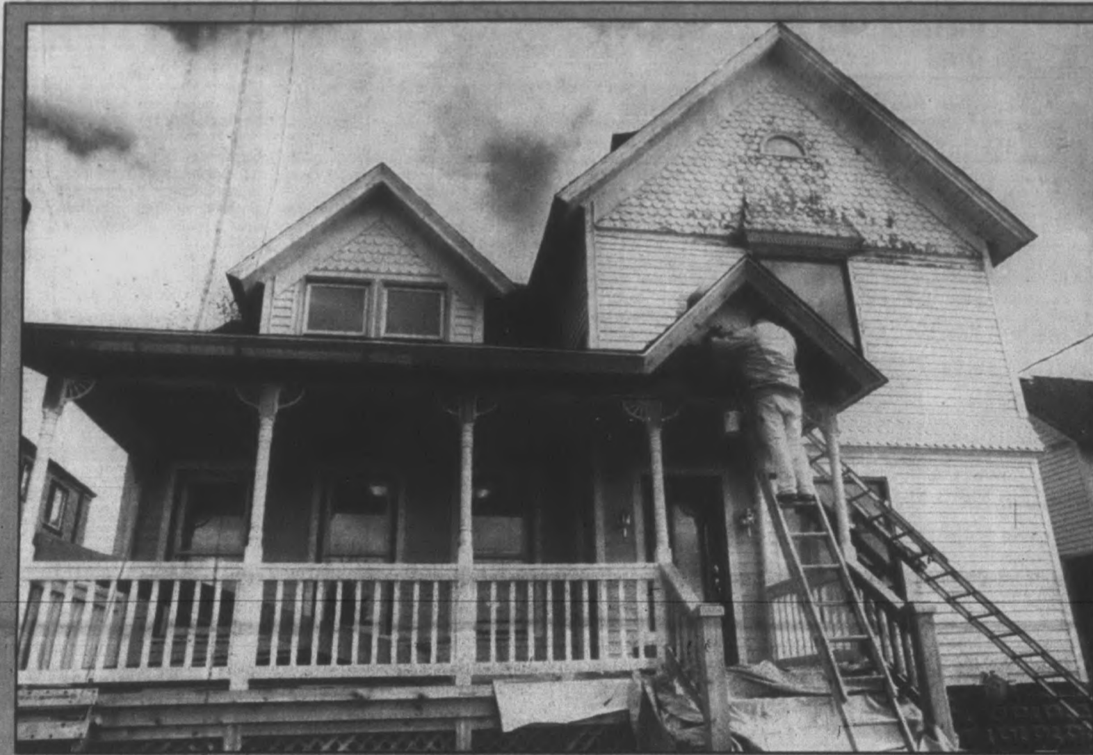
The exterior of the Johnson Investment Building in downtown Farmington is historically correct, down to the Victorian gingerbread shingles, spindles and turned posts. The
