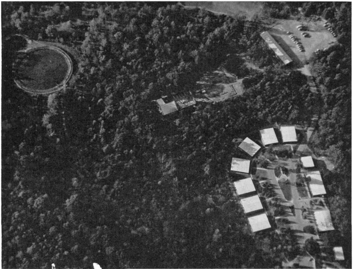
An aerial view of the Job Corps camp in Mammoth Cave Park. At lower right, portion of housing; upper right, heavy equipment and vehicle storage; center, gymnasium under construction; upper left, double sewage basin. Directly underneath the complex are some of the most extensive cave passages in the park.
