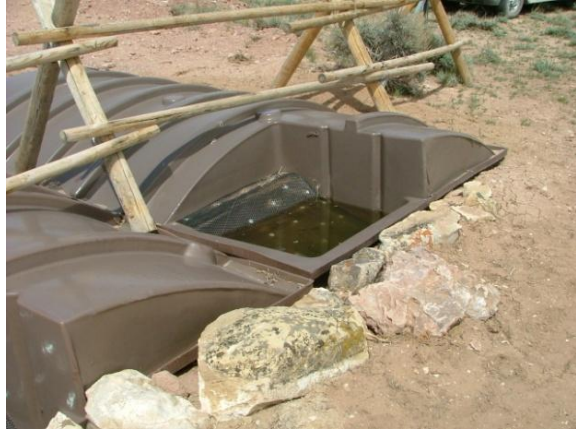
Photo 6. PMWHR “guzzler” installed in 2010 (BLM 2009).
