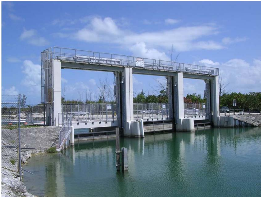
Figure 39. Water control structure (S-20F) at Mowry Canal (C-103). This adjustable weir controls water levels to the west of the park and when opened on schedule, or to relieve interior flooding, pumps large quantities of water into the nearshore of Biscayne National Park. Adjacent farms and residential areas contribute significant pollution to the canal (P. W. Harlem).
