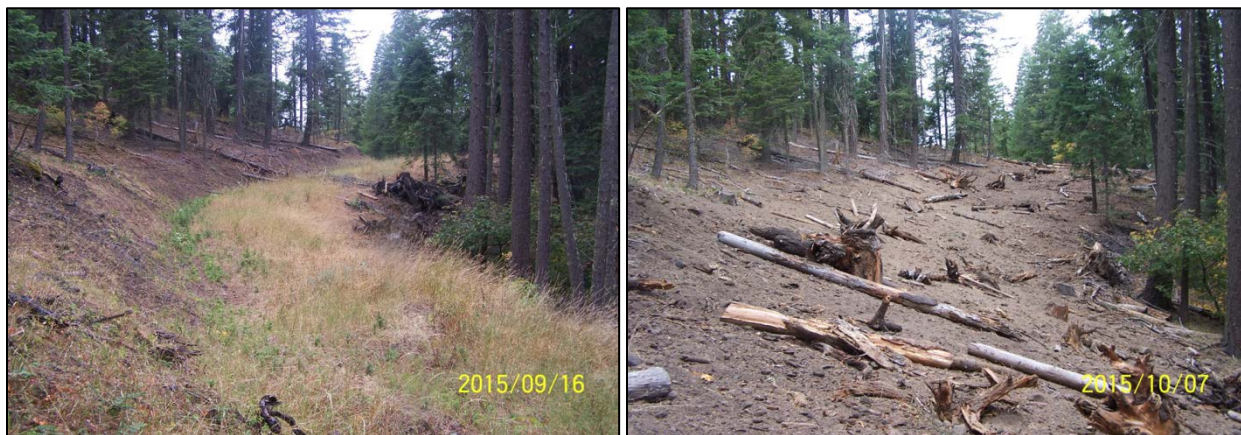
Before/After photos – road removal in the SMW
