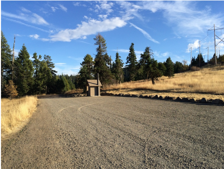
Improved parking area at Hobart Bluff trailhead with new vault toilet
