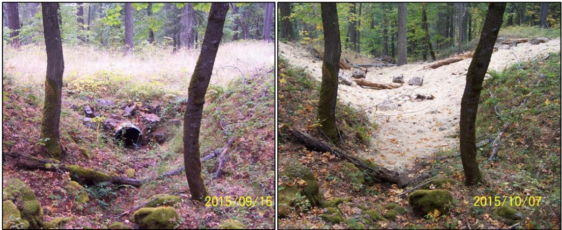
Culvert removal and restoration
