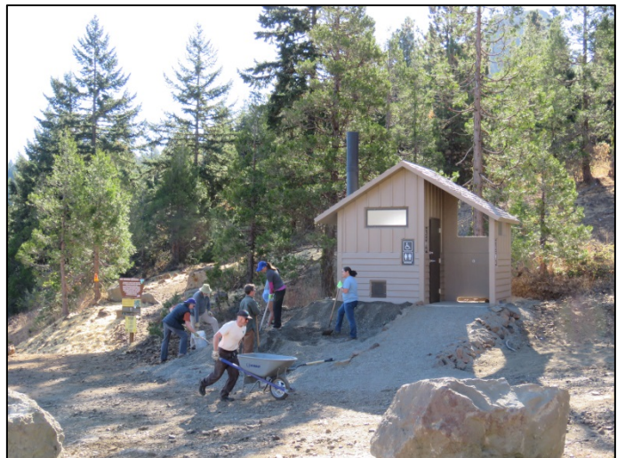
NLPD workers and new vault toilet at Pilot Rock
