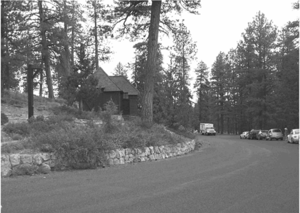
View of Lodge Access Road (2009 CLR).
