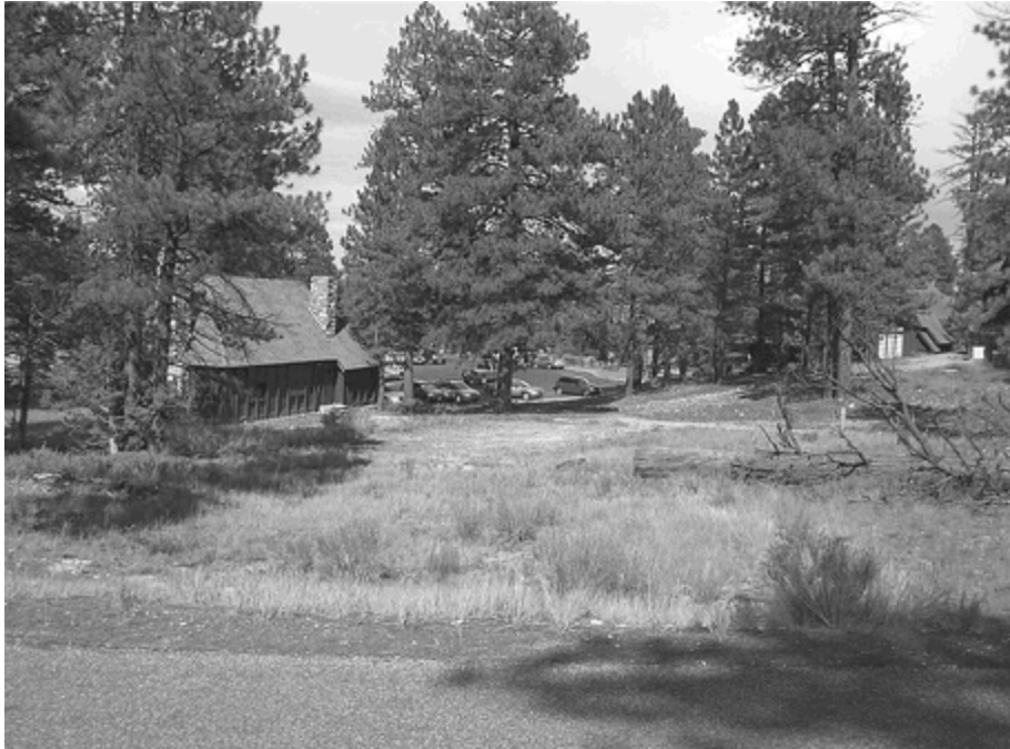
Slope between the rear of the Lodge and the dormitory buildings near the Administrative parking area (2009 CLR).
