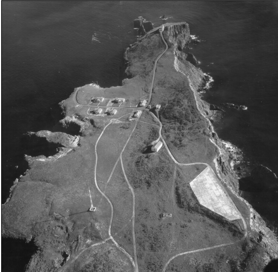
Figure 4.2.4. Aerial view of the Anacapa Light Station, December 6, 1963. Note the layout of the residences, upper left, and the rainshed, lower right. A radio tower is seen in the lower left. U. S. Navy photograph, Channel Islands National Park (Livingston 2006).
