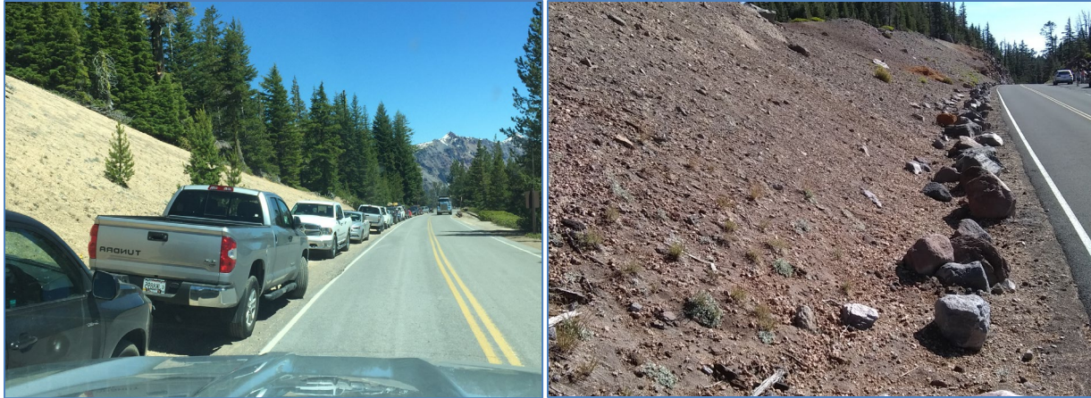
Figure 3. User-created pullouts before (left; photo by Carrie Wyler) and after (right; photo by Scott Heisler) obliteration as part of the Rim Drive Rehabilitation project.
