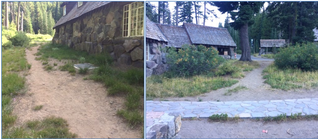
Figure 11. Large social trail created by Park staff and visitors behind the Steel VC (left) and another one in front (right). Photos by Carrie Wyler.
