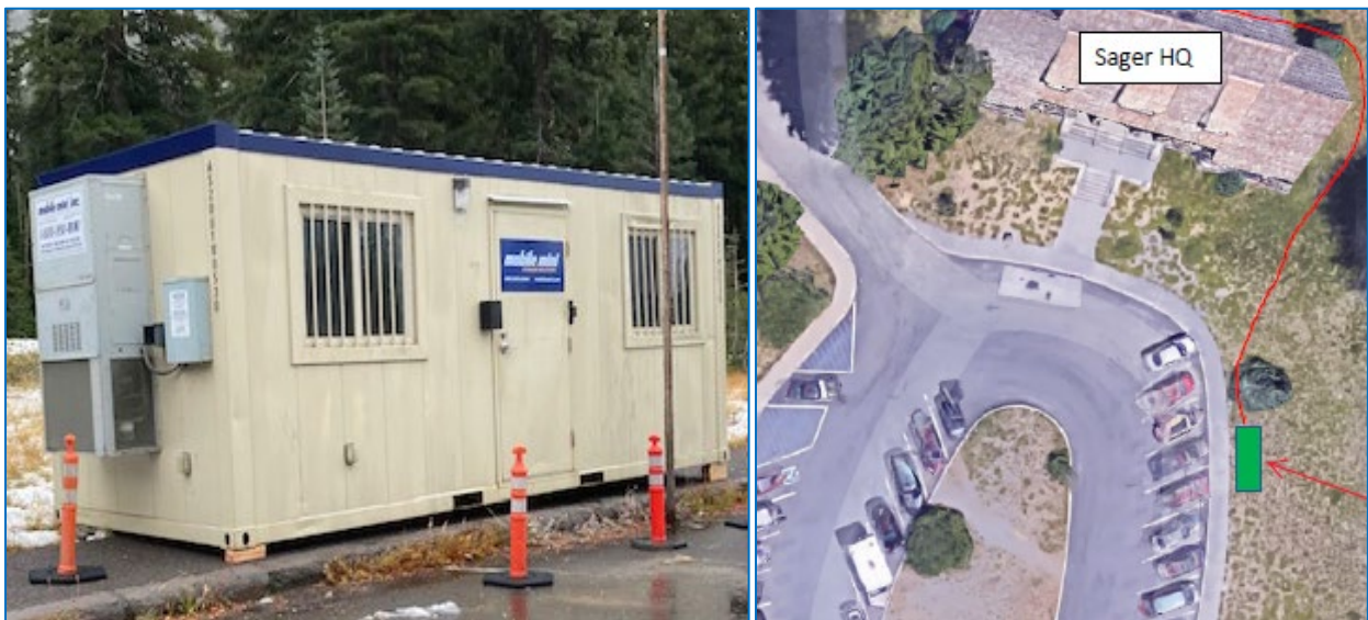
Figure 3. Temporary mobile post office structure (left -photo by Carrie Wyler) location at the headquarters parking lot (green rectangle at right – image courtesy of Ausland Group construction company).
