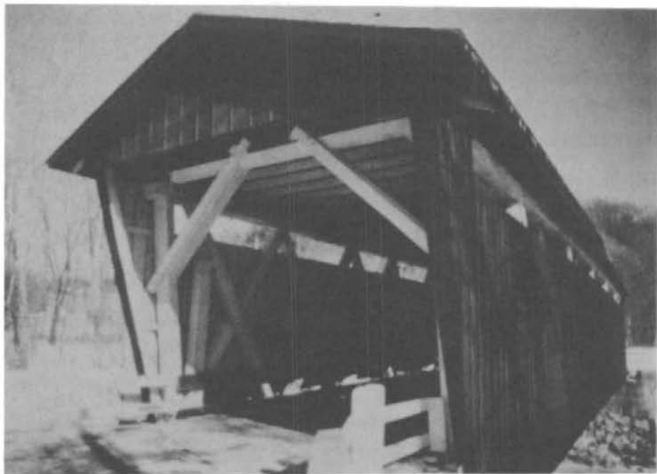
Figures 39 & 40: The 1975 wreckage (top) and the reconstructed bridge (bottom) in 1986. (Source: CRM Bulletin , June 1987)
