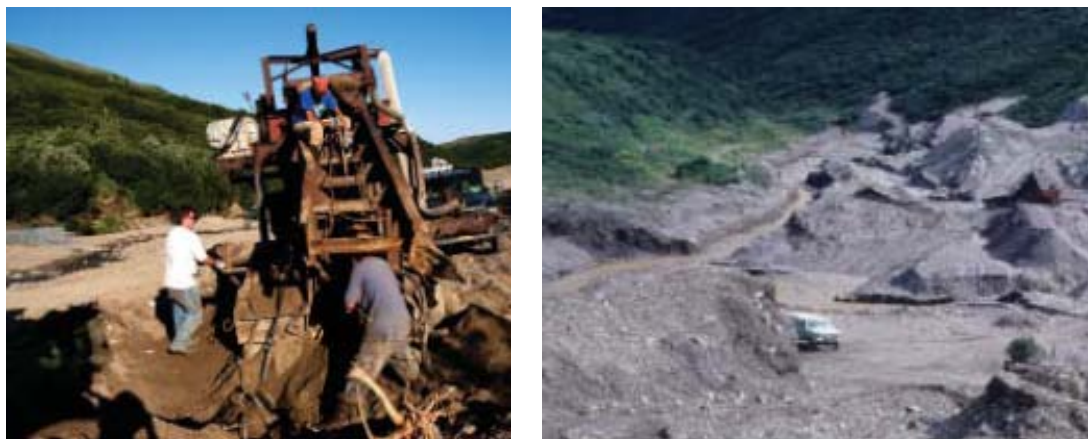
Photo B-5. Photos from Glen Creek restoration work in 2009: removing abandoned mining debris (left) and tailing piles to be leveled (right) (NPS photos, in DENA 2010b).
