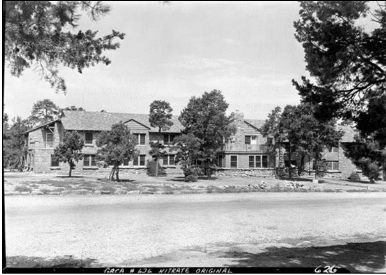
Figure 16. Victor Hall, 1936. The Fred Harvey Company's men's dormitory in Grand Canyon Village, designed by architect Mary Colter (NPS photo).
