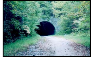
Tunnel at end of Lake View Road constructed in 1970.
