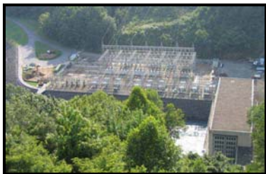
Fontana Reservoir provides 300 MW of electrical generating capacity.
