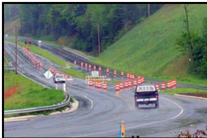
Widening of NC 28 to four lanes
