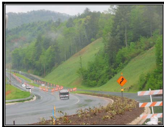
Construction on NC 28, Summer 2003
