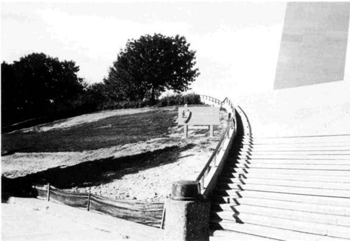
Figure 68: View of Grand Staircase from Leonor K. Sullivan Boulevard, (Bellavia, 1995).
