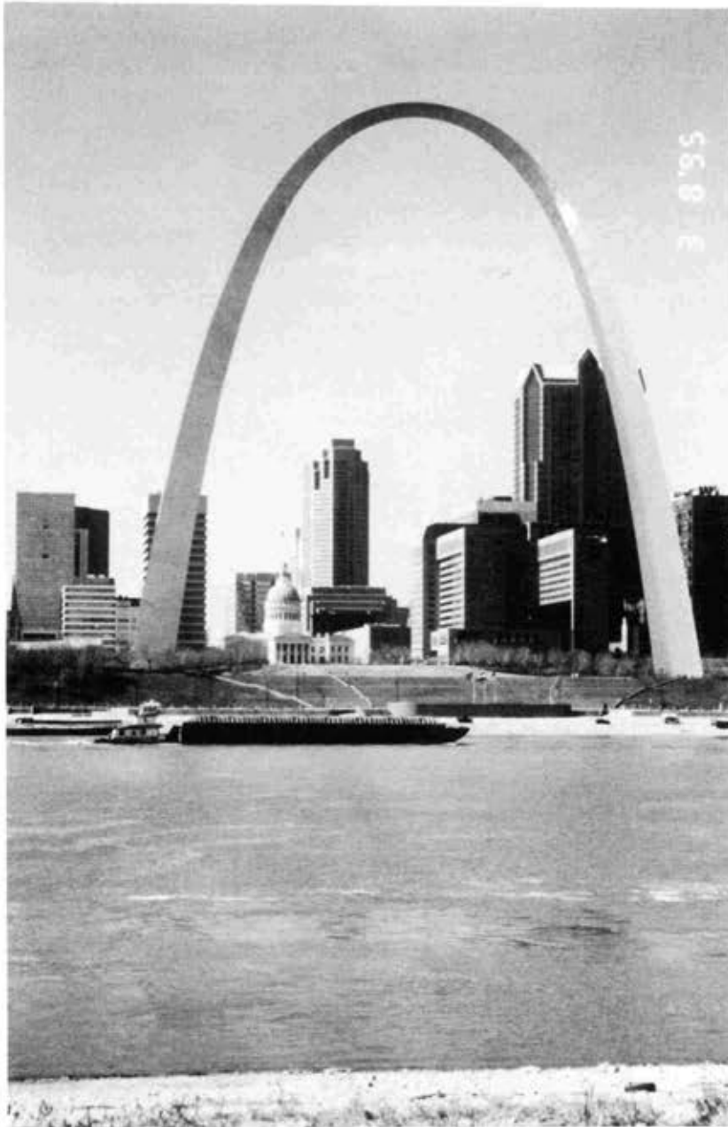
Figure 83: View from East St. Louis toward Gateway Arch. (Bellavia, 1995).
