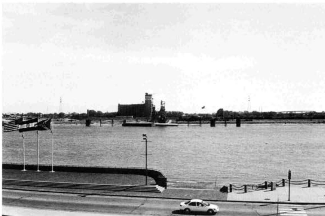
Figure 54: View of Continental Grain Elevator across from the Arch, (Bellavia, 1995).
