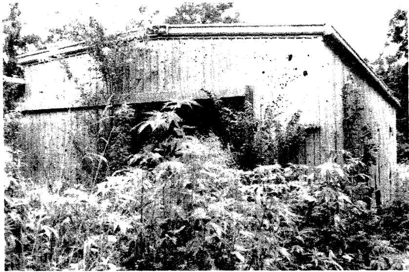
Photo 19. Illegal Pumphouse, Barataria District.
