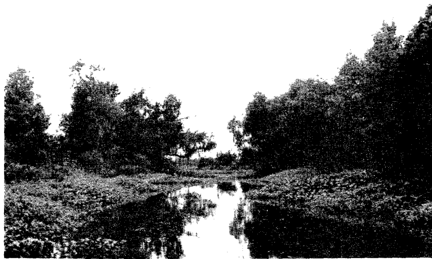
Photo 20. Powerline, Barataria District.
