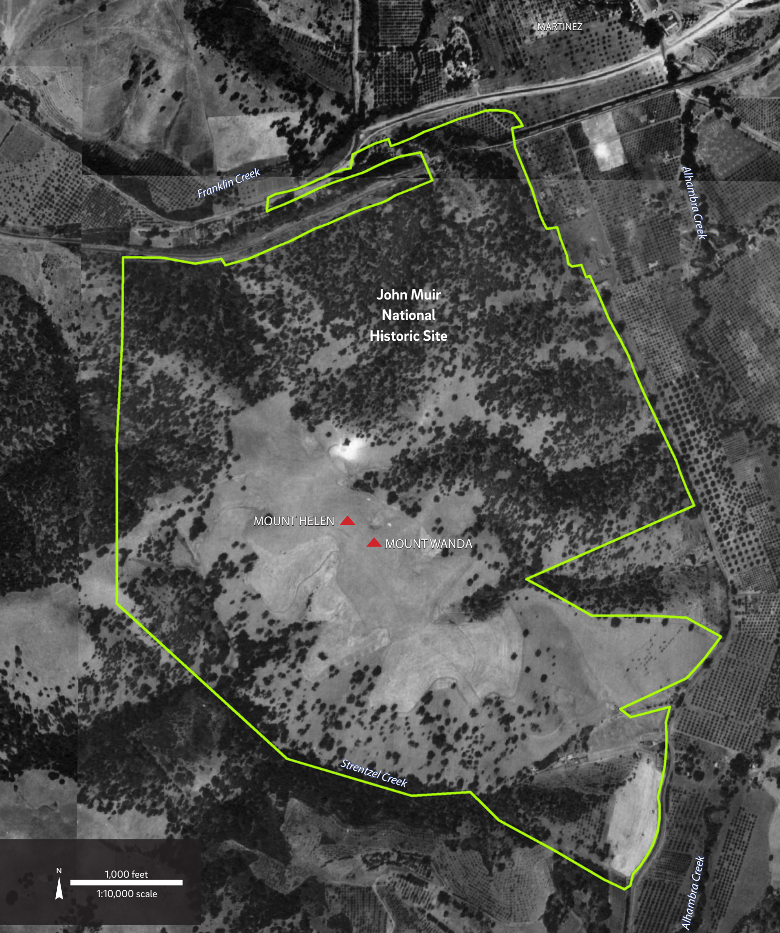
Figure 21. The Mt. Wanda landscape visible in the 1939 aerial photographs appears to reflect the same general ecological patterns documented in 19th century sources. Forests and woodlands cover the northern and southernmost portions of the study area, while grasslands and oak savanna occupy the central, higher-elevation portions. (USDA 1939)
