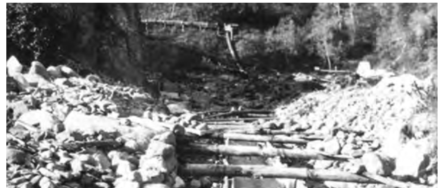
Bowman’s placer operation on Portage Creek c. 1937 with flume, penstock, hydraulic giant, and diversion channel – technologies used widely throughout the region. H-334, courtesy of Howard and Letitia Bowman.
