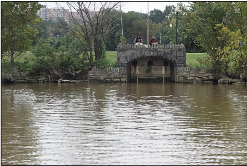
Perfect fishing site on the Anacostia River, an abandoned CSO outfall from the 1930s. November 2018 (Anacostia Park). Photo credit: S.J. Fiske
