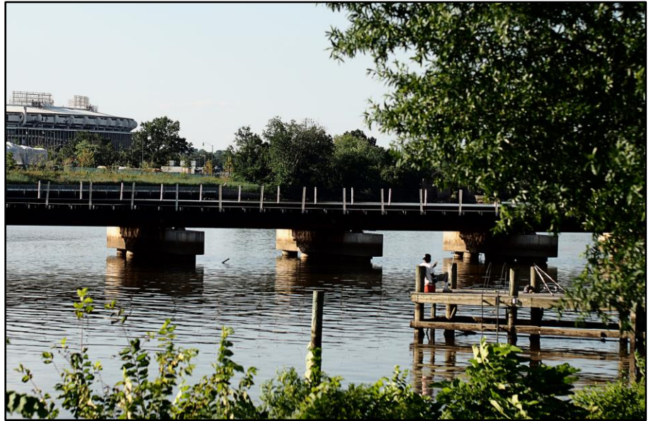
Favorite spot on the Anacostia; RFK Stadium and CSX rail bridge in background. Photo credit: J. Trombley
