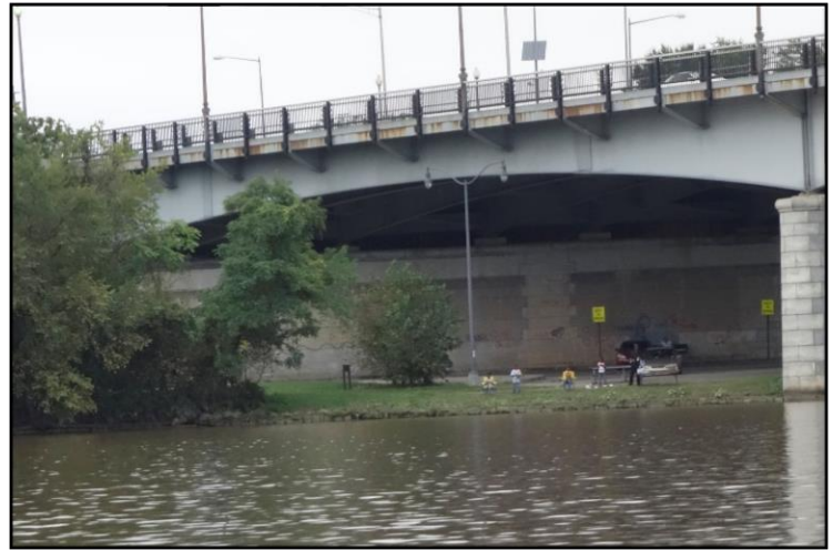
Fishing under the Pennsylvania Street Bridge, November. Photo credit: S.J. Fiske
