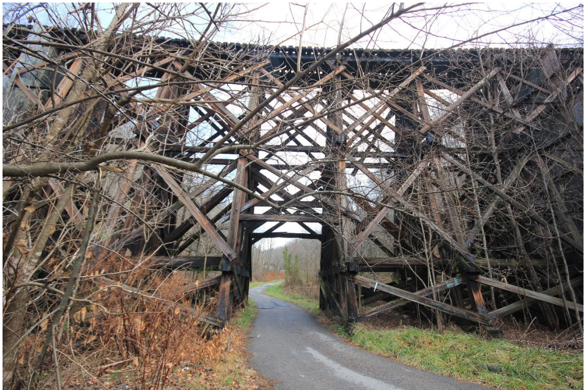
10. Railroad resource: Jenkinjones Norfolk & Western trestle. (MD-0876)
