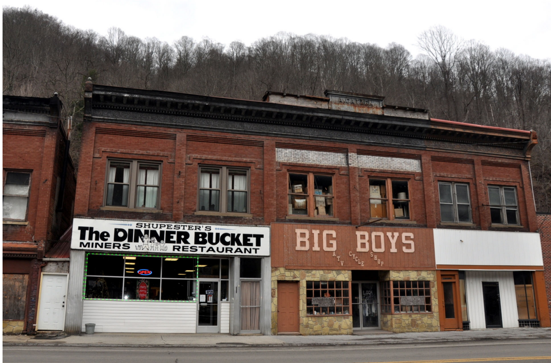
12. Commercial buildings, Northfork historic district. (MD-0608)
