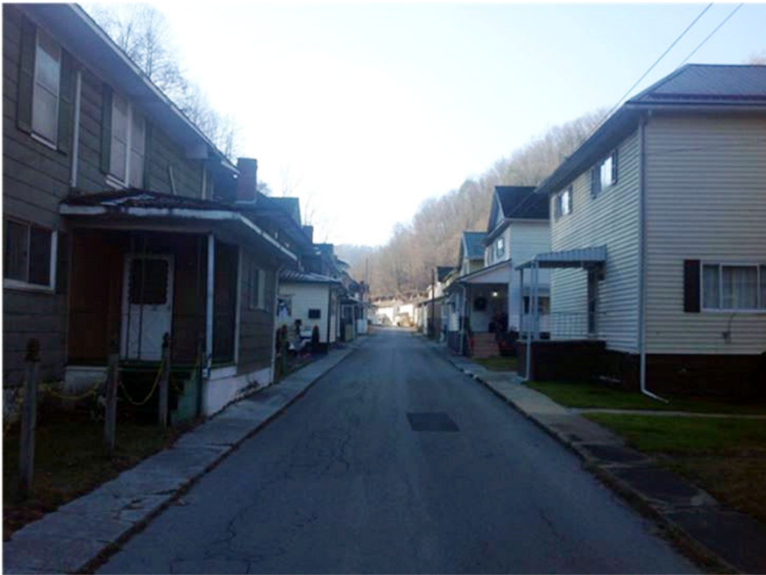
4. Filbert streetscape with long, narrow houses.
