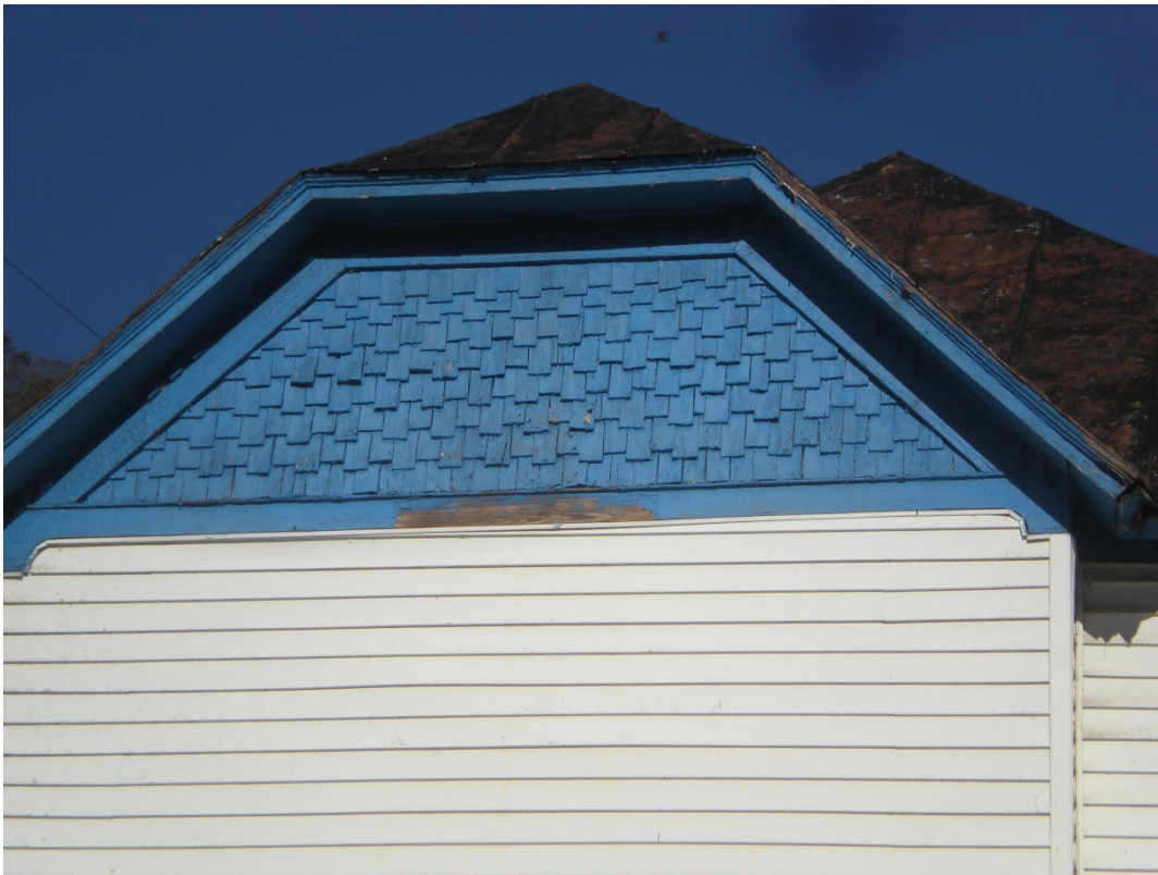
8. Jerkinhead roof, wood shingles, vinyl siding: original architectural features and alterations.
