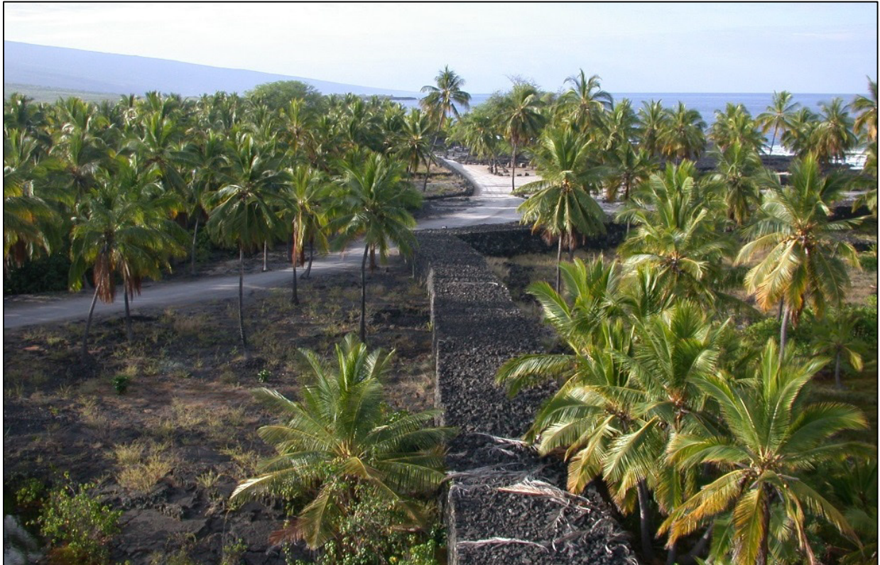
Figure 2.2-1. The Great Wall, bounding the south and east sides of the Pu‘uhonua (place of refuge; NPS photo).
