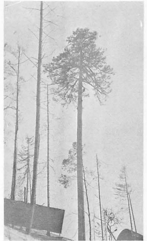
HIGH CLIMBER JUST BELOW THE CROWN OF THE DOUGLAS FIR TREE READY TO TOP THIS TREE FOR A SPAR TREE IN HIGH LEAD LOGGING, FORT BRAGG, June 1925
