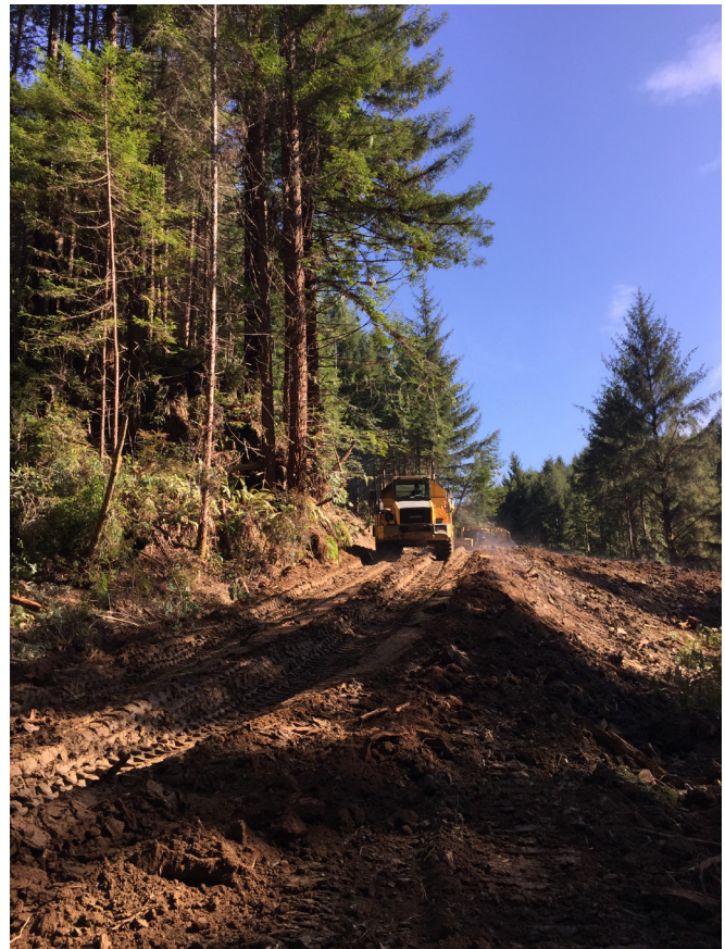
Figure 23. Photograph of restoration activity along Lost Man Creek. In the Redwood Creek watershed, Lost Man Creek flows into Prairie Creek, which flows into Redwood Creek. The Franciscan Complex coherent unit of Lacks Creek (KJfl) underlies the Lost Man Creek basin. Like restoration activities elsewhere in the parks, road removal here required the use of heavy equipment to excavate stream-crossing fill material, restore channels close to their original configuration, and place excavated fill in stable locations to best mimic pre-disturbance topography and drainage patterns. Photograph by Katie KellerLynn (Colorado State University), taken 8 October 2019.
