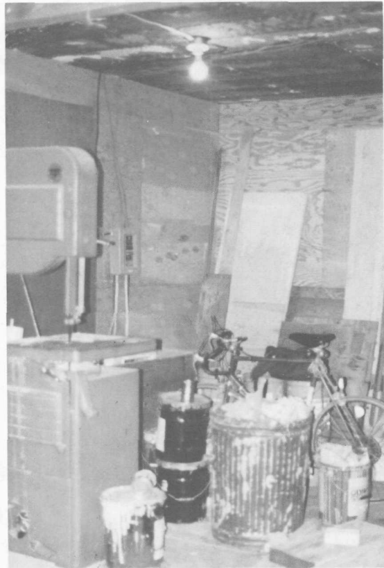
FIGURE 25. North room, northwest corner.
