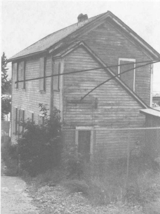
FIGURE 20. View from northeast.
