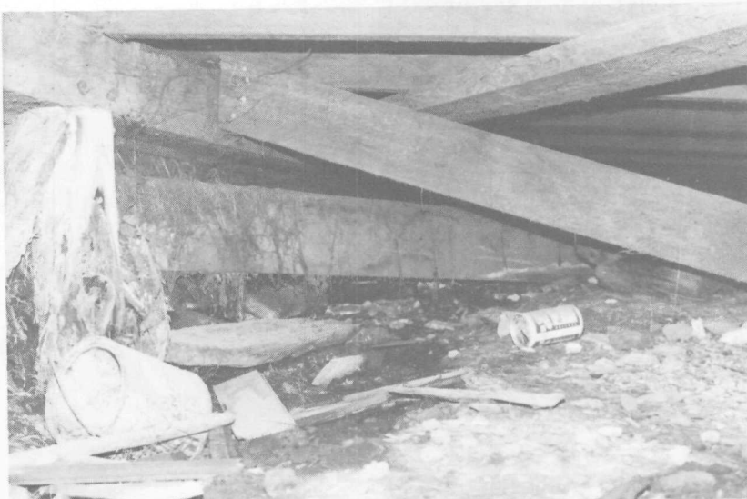
FIGURE 31. Crawl space, west side of building.
