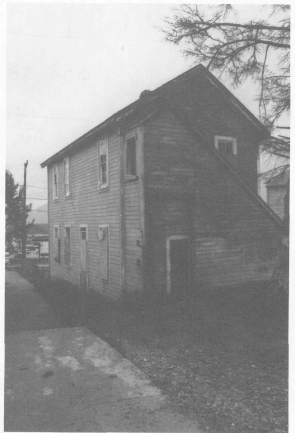
FIGURE 14. View from northeast.
