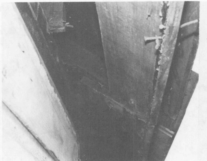
FIGURE 19. Soffit at west eave.
