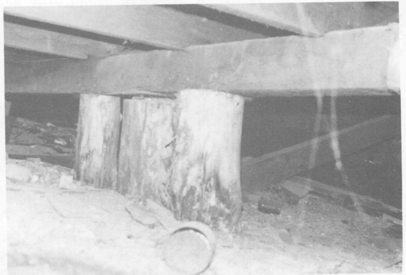
FIGURE 30. Crawl space, east side of building.
