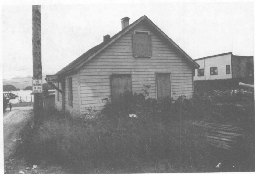
FIGURE 9. View from northeast.
