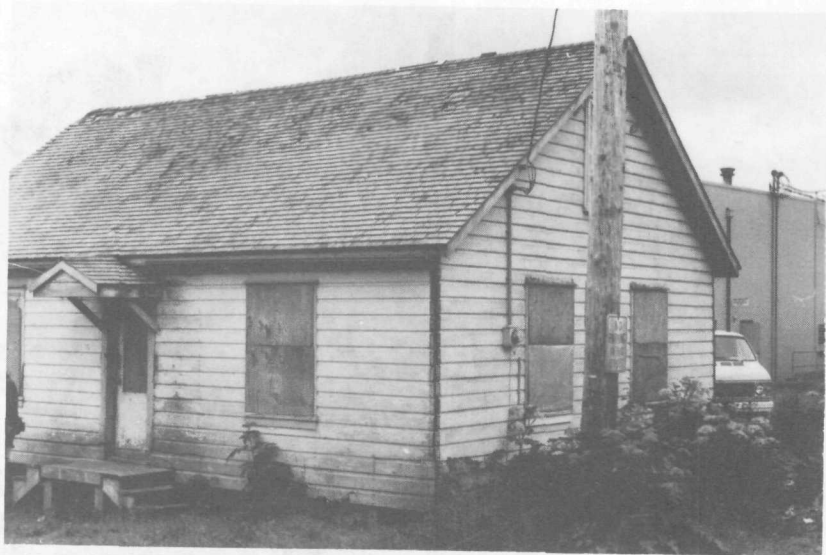
FIGURE 11. View from northeast.
