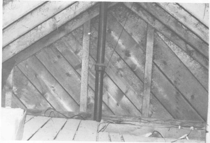
FIGURE 32. Attic, north end.
