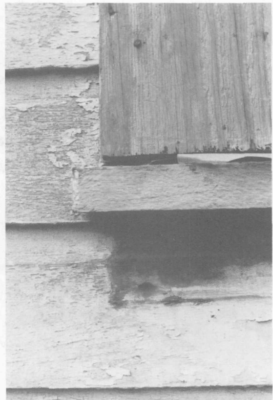
FIGURE 16. Paint ghost detail indicating found trim is original.
