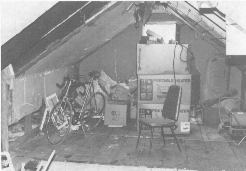
FIGURE 30. Attic, northwest corner.
