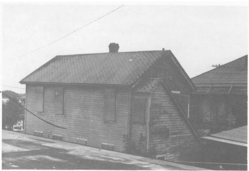
FIGURE 19. View from northeast.
