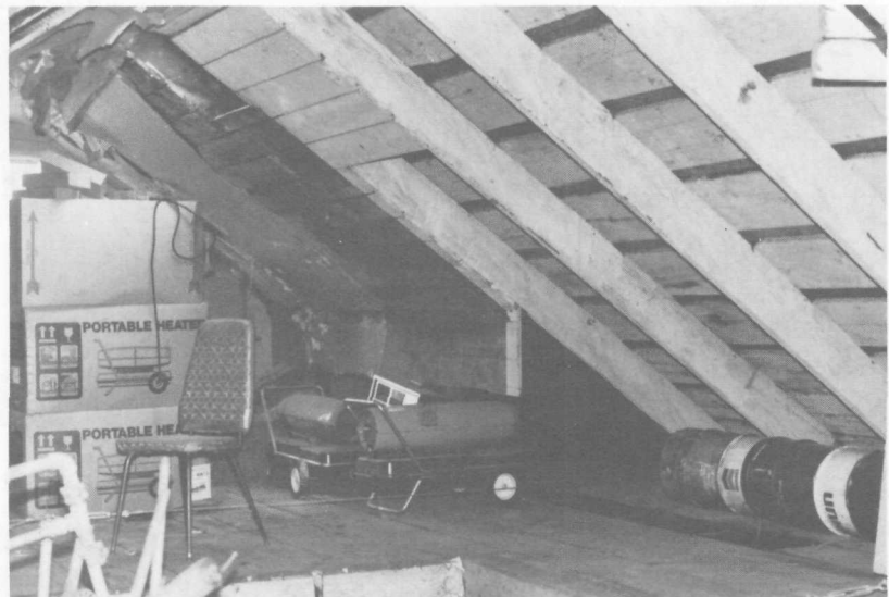
FIGURE 31. Attic, northeast corner.
