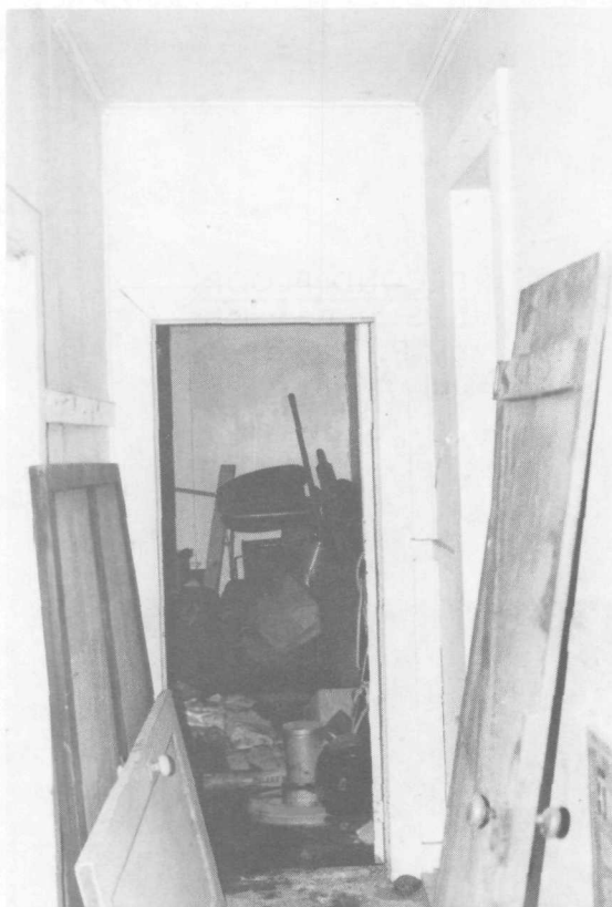
FIGURE 34. First floor, west hallway, south end.
