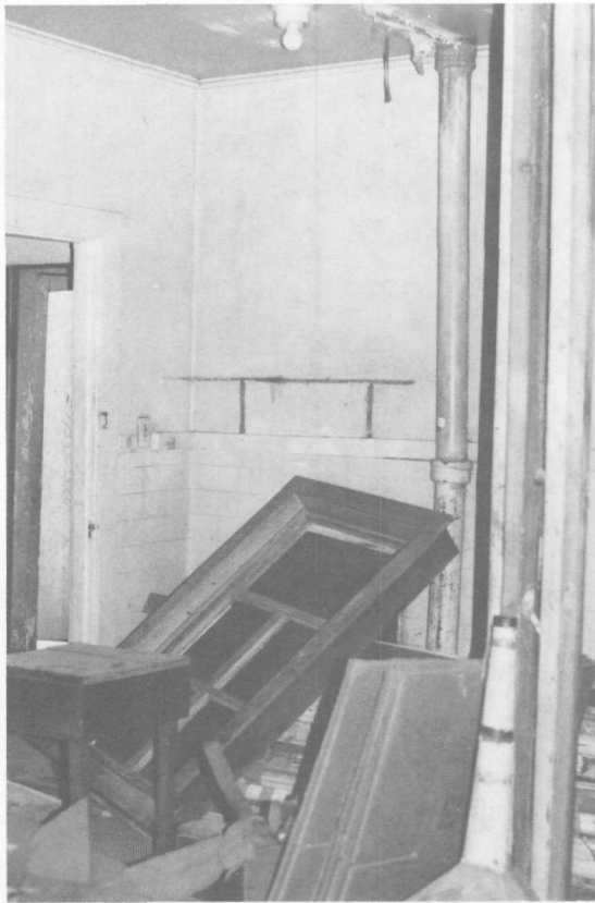
FIGURE 45. Northwest corner, northeast room, first floor.
