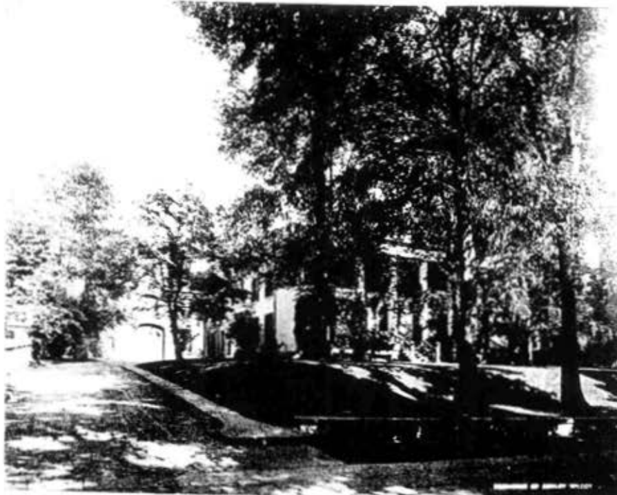
Figure 1.23. Northwest corner, seen from Delaware Avenue, circa 1896-1906.
