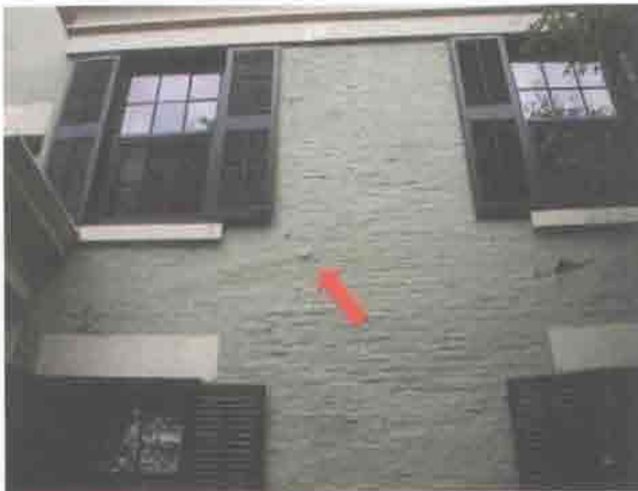
Figure 2.14. North elevation, detail of brickwork scars from formerly attached barracks building.
