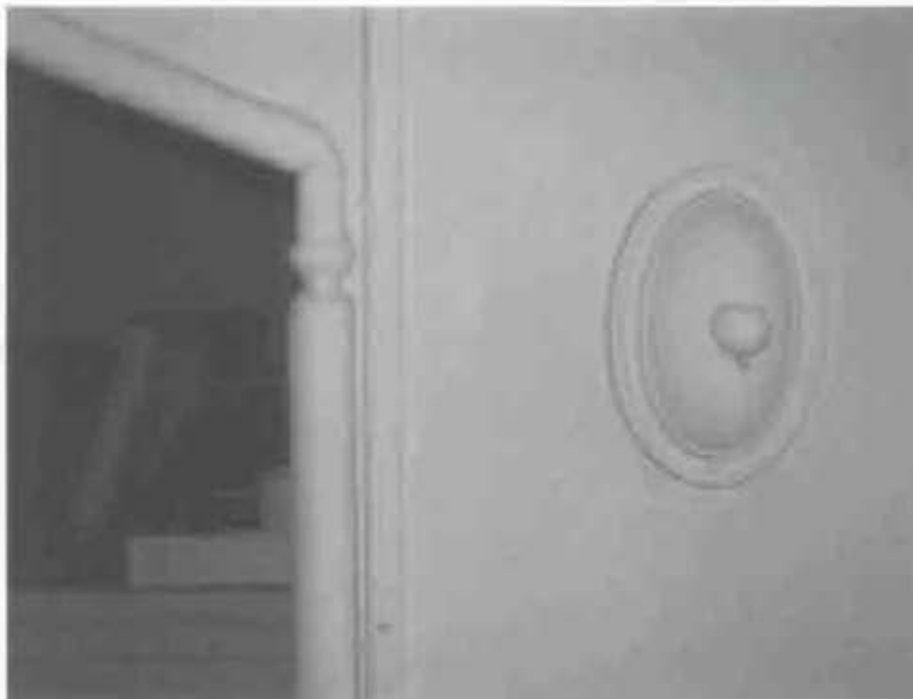
Figure 2.81. Room 306, wood corner guard on edge of recess, and remnant of light fixture.
