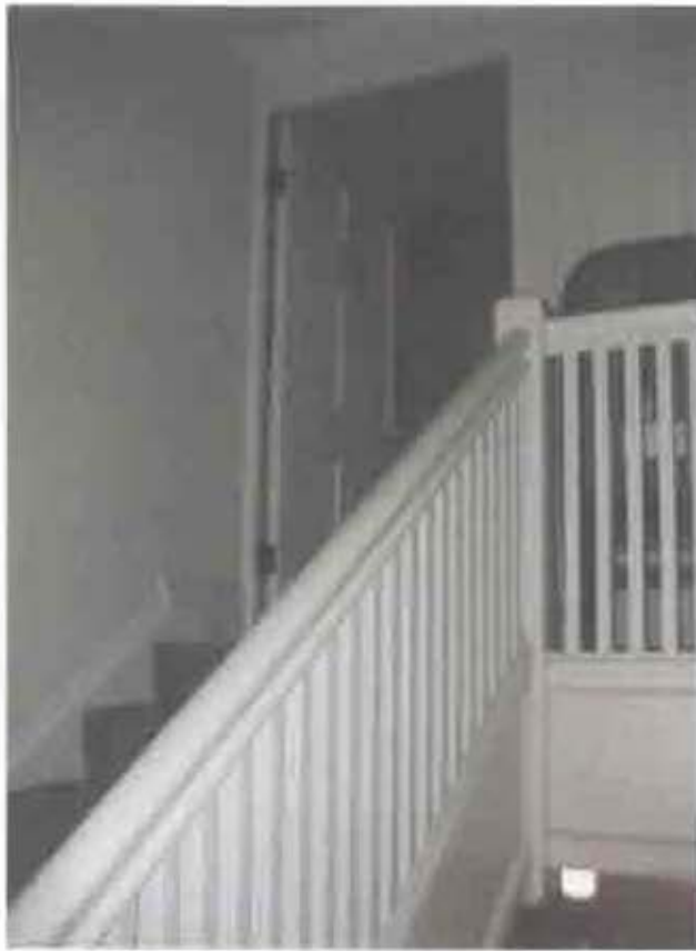
Figure 2.72. Room 301 (North Staircase).
