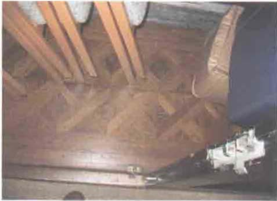
Figure 2.30. Room 101 (Vestibule), ca. - 1885 parquet flooring.
