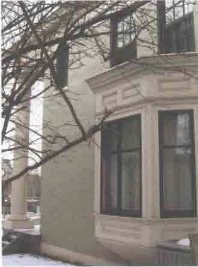
Figure 2.1. South elevation, west end of original building.
