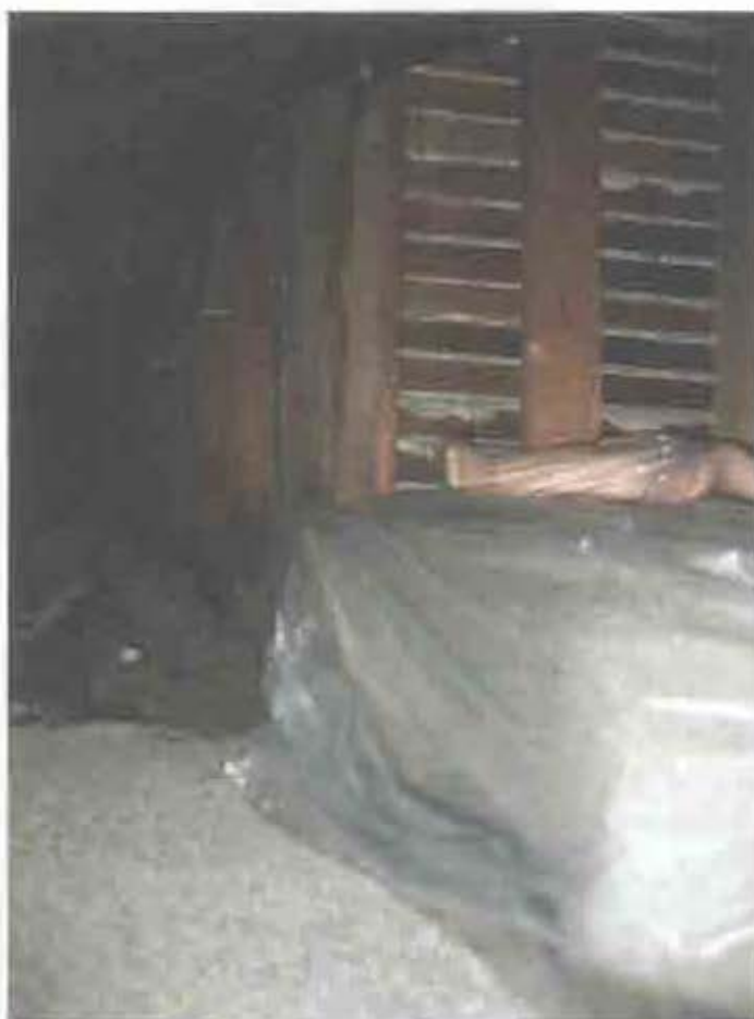
Figure 2.71. Room 308a, looking west toward dormer check wall.
