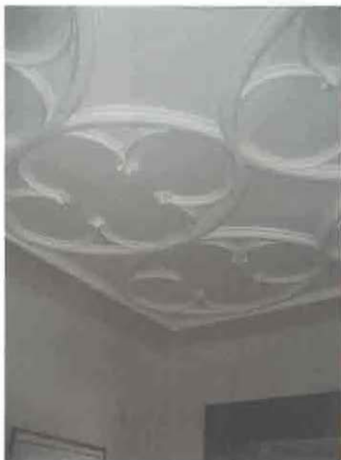
Figure 2.41. Room 107 (Living Room), ceiling.
