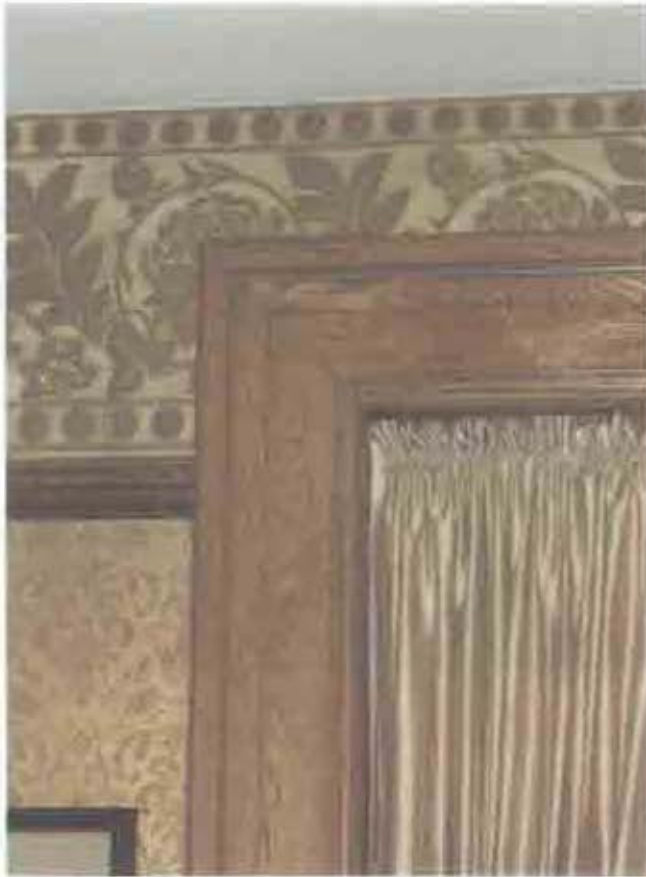
Figure 2.34. Room 104 (Library), molded oak casing.
