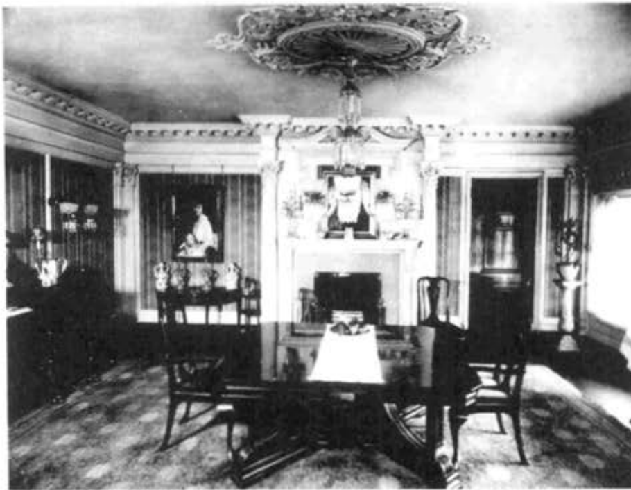
Figure 1.46. Dining Room (room 108), looking east, circa 1921.
