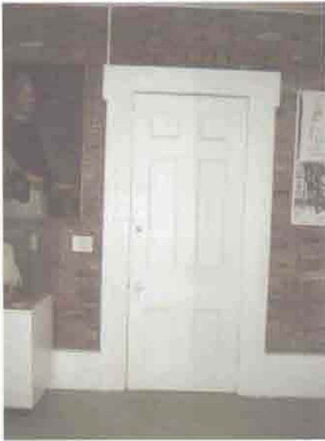
Figure 2.54. Room 203 (Second-Story Back Hall), west wall, pre-1938 doorway and brick infill.
