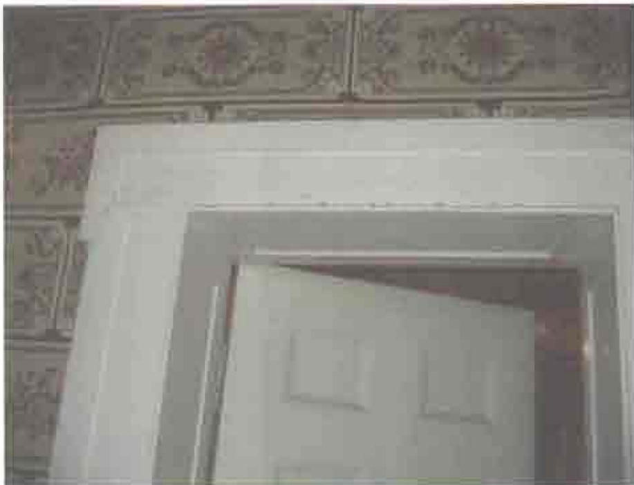
Figure 2.55. Room 201 (Second-Story Stair Hall), pre-1938 doorway.
