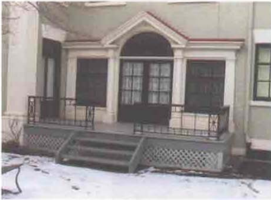
Figure 2.5. South elevation, Dining Room porch.
