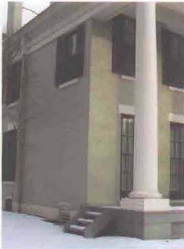
Figure 2.6. Northwest corner of original building.
