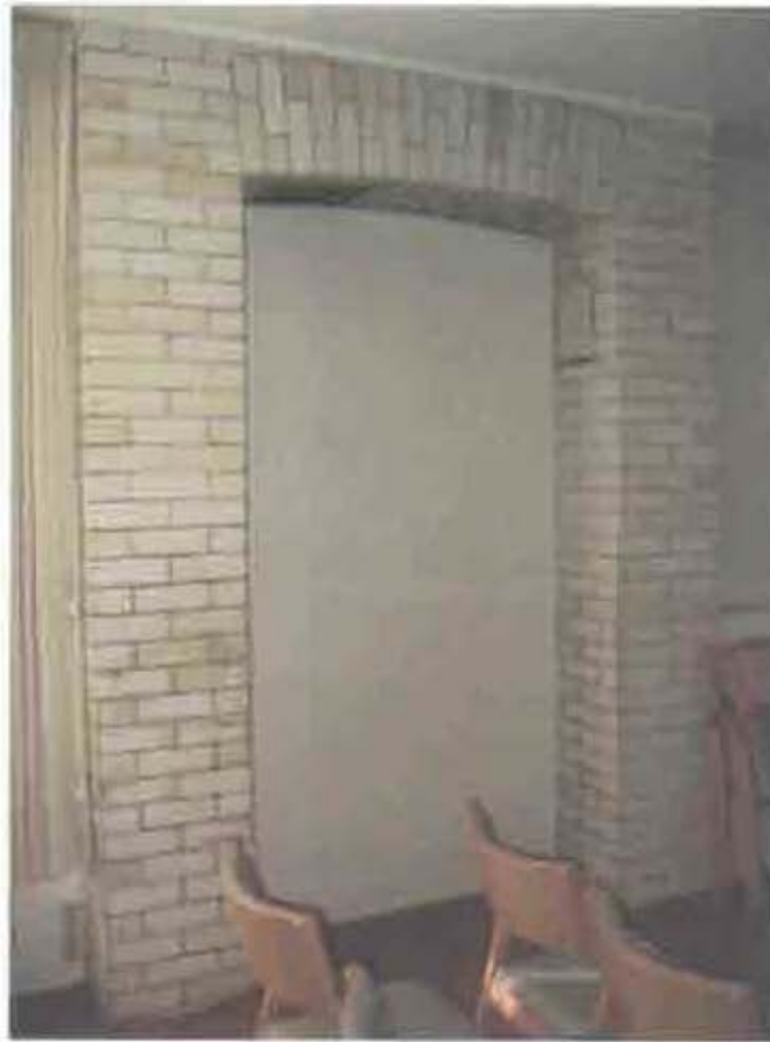
Figure 2.48: Room 112 (Kitchen), fireplace.
