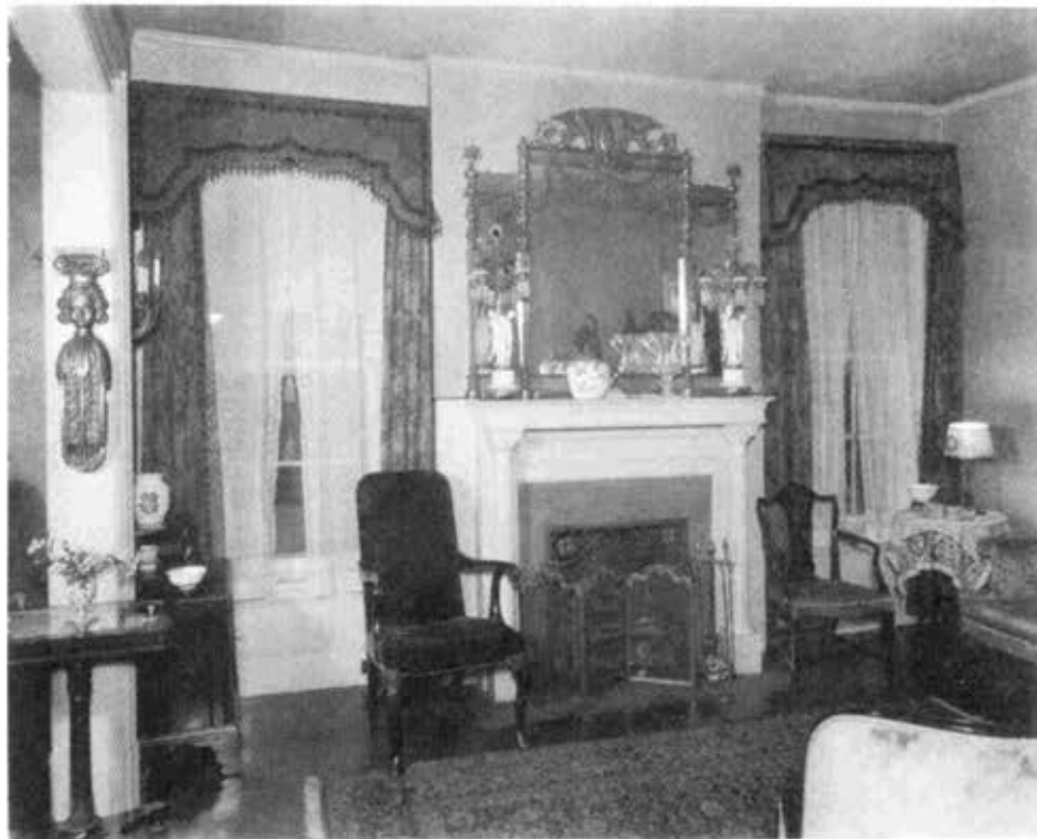
Figure 1.43. East half of Double Parlor (room 103), north wall, circa 1921.
