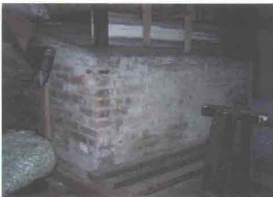
Figure 2.17. Room 001, north retaining wall.
