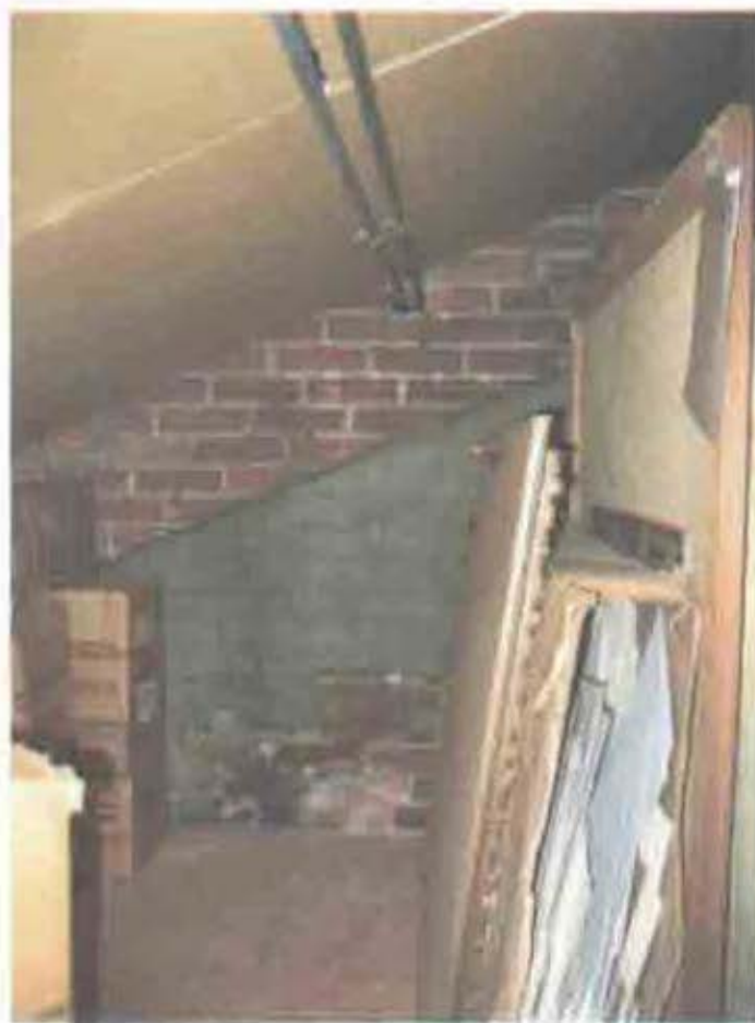
Figure 2.82. Room 307, looking west toward original brick gable end wall, showing roof line of 1864- 1865 addition and paint evidence.
