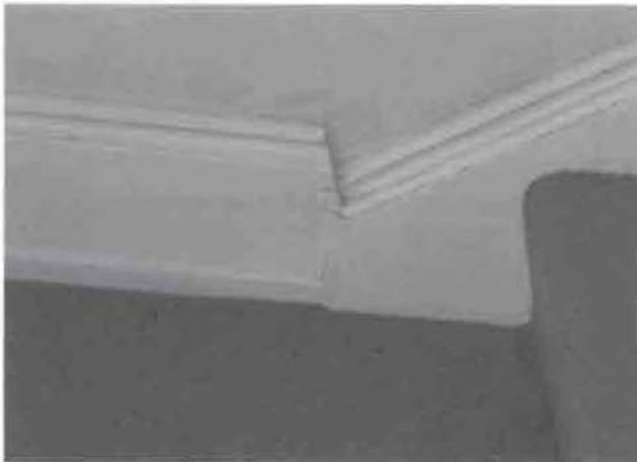
Figure 2.73. Room 301 (North Staircase), baseboard.
