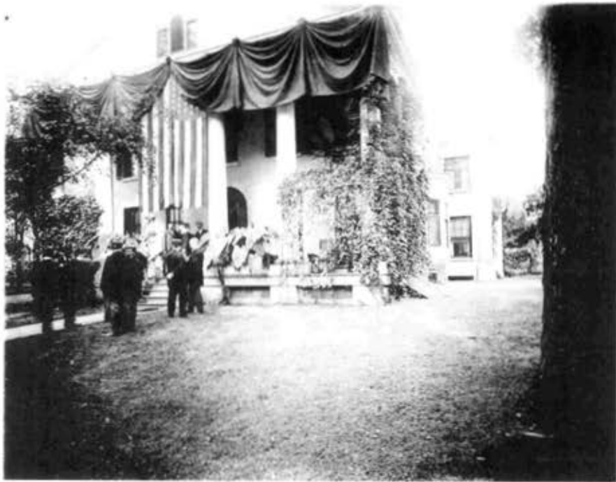
Figure 1.19. "West facade, September 14, 1901 - I."
