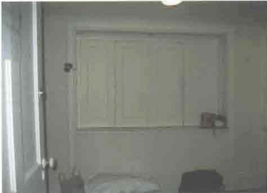
Figure 2.75. Room 302 (Hall), south- wall linen closet.
