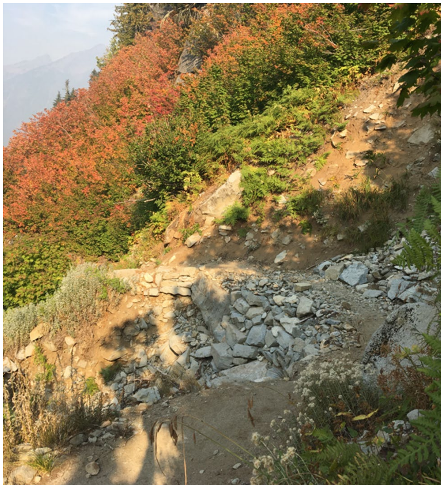
Figure 2. Intermittent stream crossing best management practice in place along a section of the PNT in the North Cascades.
