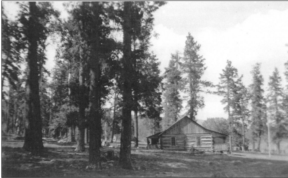
Figure 5.9. The Ranch Foreman's House, also known as the Manager's Cabin, was (like the Bond Cabin) built in 1918. This photo was taken before the south wing was added.
