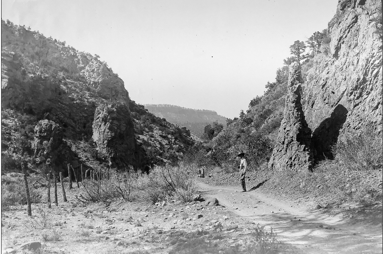
Figure 4.2. The unimproved condition of the Jemez Springs Road is shown in this 1910 photograph. Photo courtesy of: New Mexico State University Library, Archives and Special Collections, Image 01030327.
