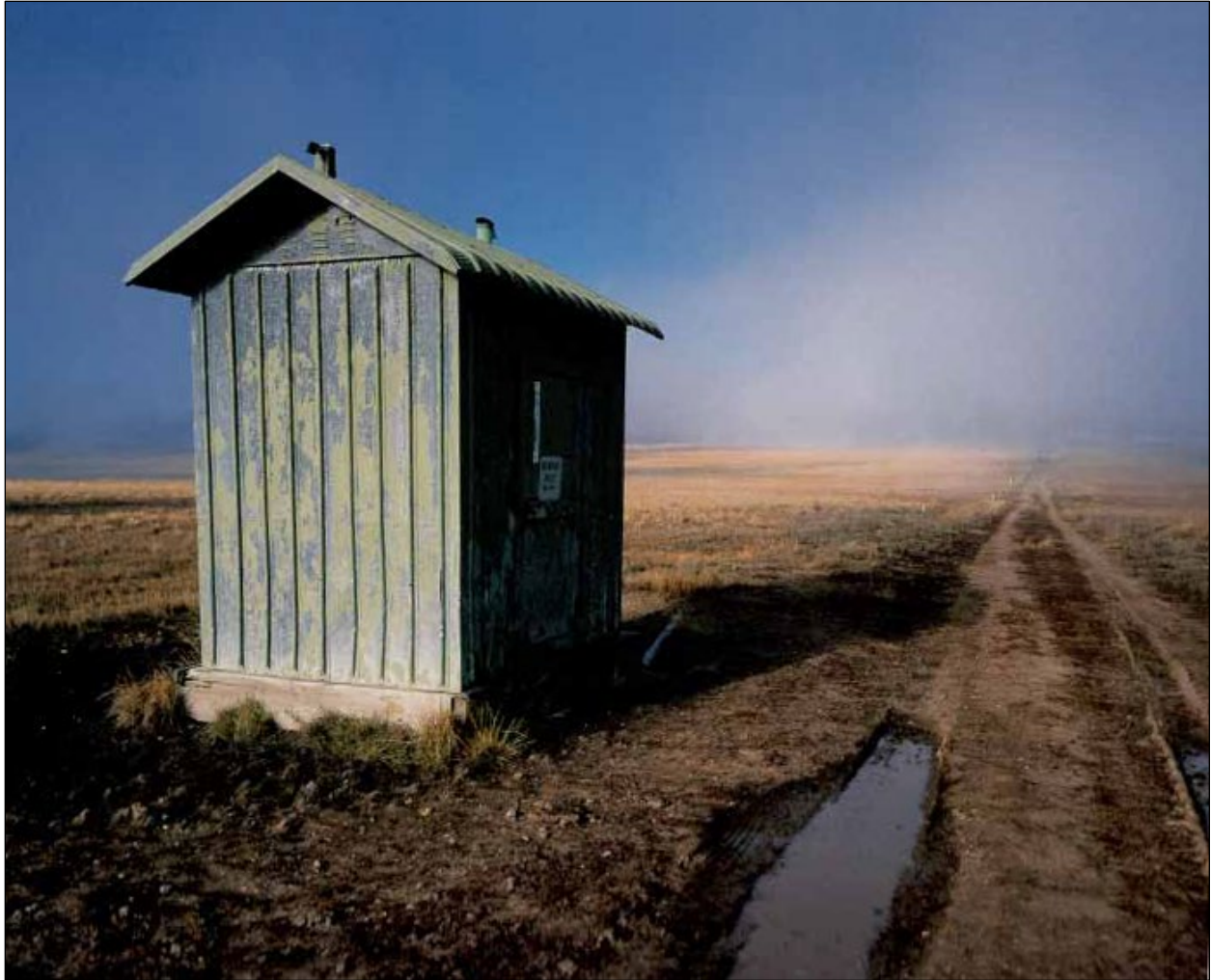
Figure 4.14. In 1949–1950, the Atomic Energy Commission constructed a gas pipeline across the Baca Ranch. Shown here is a maintenance road along its right-of-way, together with a small maintenance facility. Natural gas pipeline road and shack, Valle San Antonio, 2005. Photograph by Don J. Usner. From Valles Caldera: A Vision for New Mexico's National Preserve , 1st ed., William DeBuys and Don J. Usner (Museum of New Mexico Press, 2006). Courtesy of the publisher.
