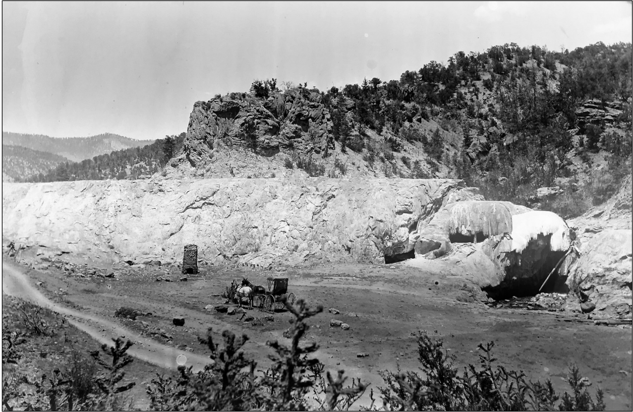
Figure 4.1. This photograph of the Soda Dam, taken in 1910, shows the Jemez Springs Road in the foreground. Photo courtesy of: New Mexico State University Library, Archives and Special Collections, Image 01030349.
