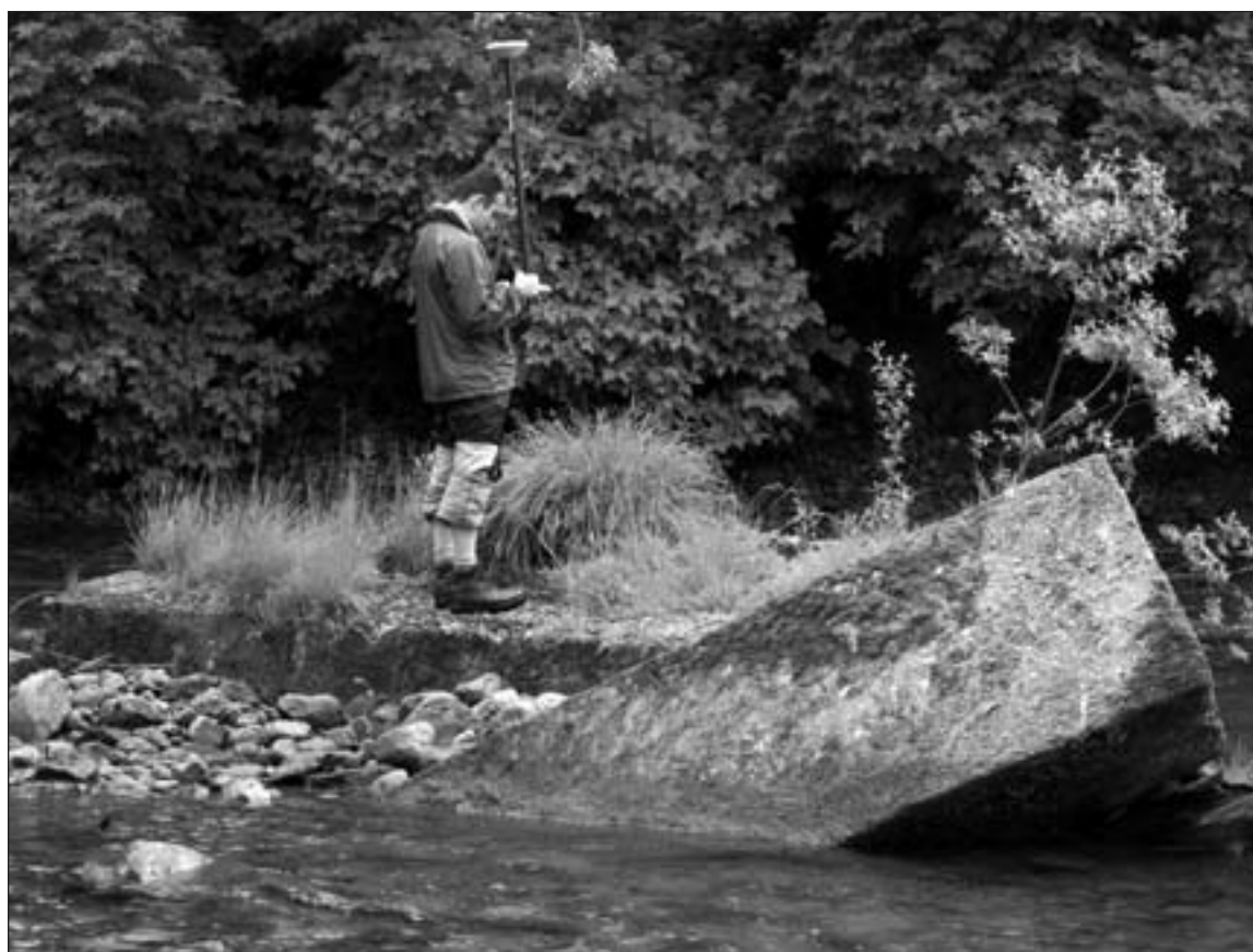
Figure 5-36. Concrete bridge abutments in the Indian River.
