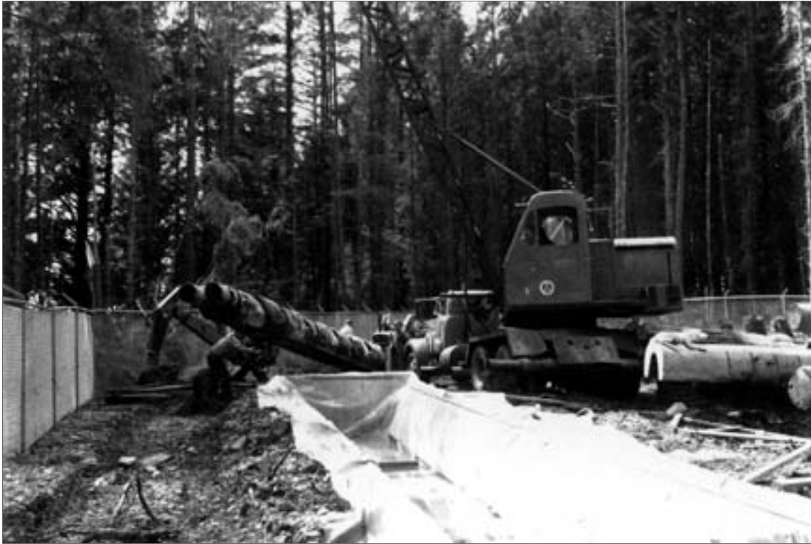
Figure 2-12. Dipping the park's totem poles in a Fort Clearing trench of preservative, 1972 (courtesy Sitka National Historical Park).
