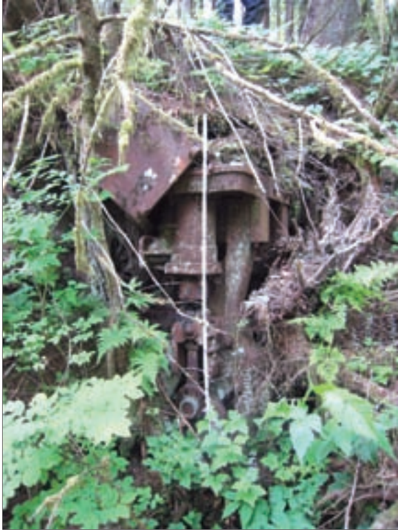
Figure 9-2. Cast iron water pump casing in the west bank of the Indian River.
