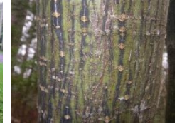
F - Stripes > Vert. Crack
