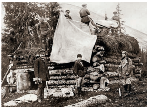
Photo 3. The first "skyscraper" in Khibiny built by V.I. Vladavets exploration crew (Vortkeuai River valley at the Kukisvumchorr bottom). 1928.
