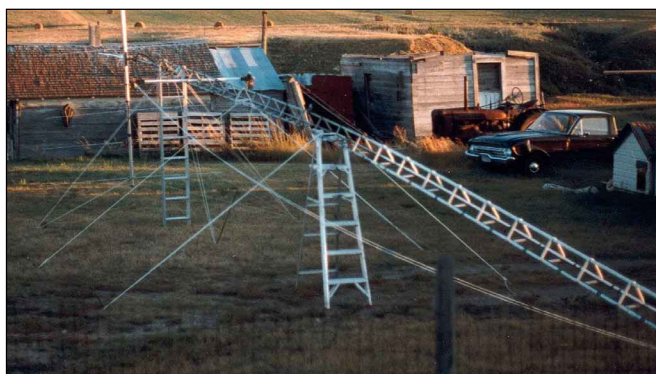
They're accustomed to high winds in northeastern Montana. K7SAM needed to work on his 50-foot fold-over tower, so he decided to tie it down securely. When the "breezes" can gust to 75 MPH, even a horizontal tower can take flight!
