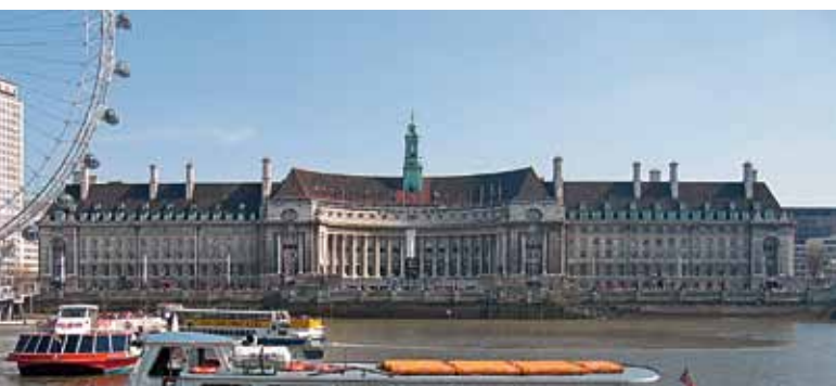
Fig. 8: ex County Hall 1911–22 and 1931–33, Ralph Knott, Westminster Bridge SE1 Built as headquarters of London County Council, now hotel. Island site with frontage to Thames; six storeys plus two in huge roof, planned round multiple light-wells. Steel frame, Portland stone cladding
