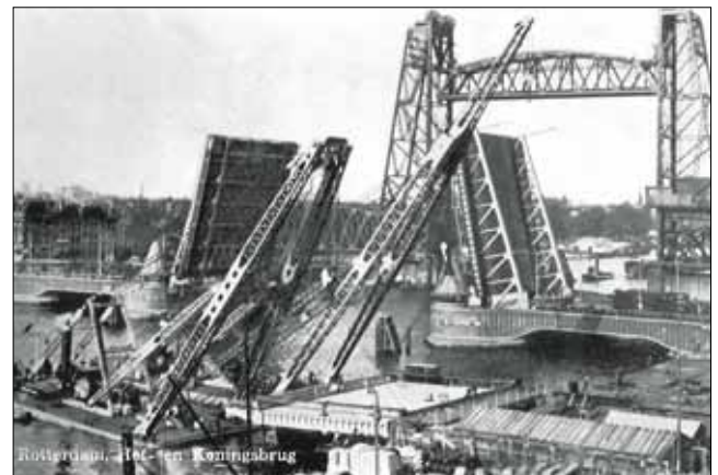
Figure 6: De Hef and the Koningsbrug, two bridges in the Koningshaven
