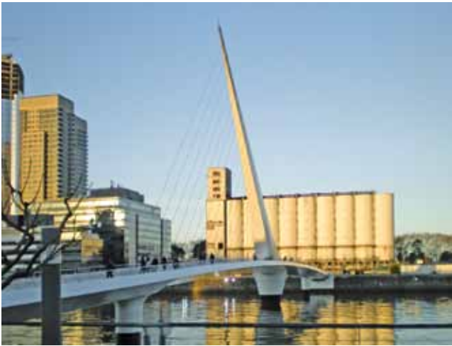
Figure 12: Bridge by Santiago Calatrava
