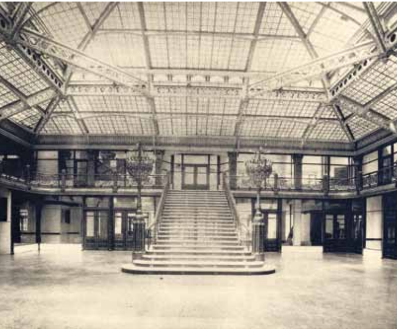
Figure 8: Interior, The Rookery (1885–1888), Chicago, Burnham & Root
