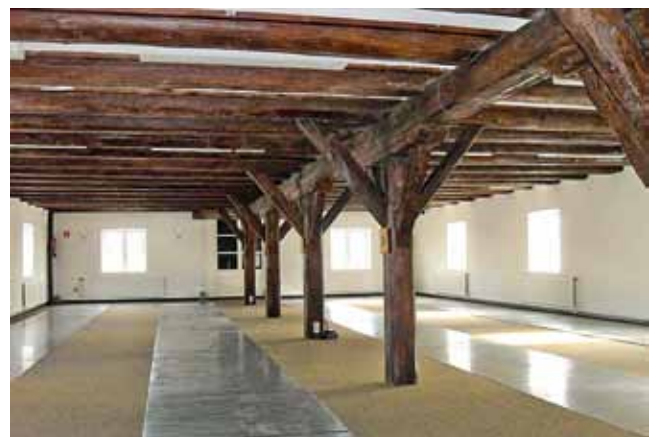
Abb. 5: Bremen, Vegesack, Thiele-Speicher um 1800, innen
