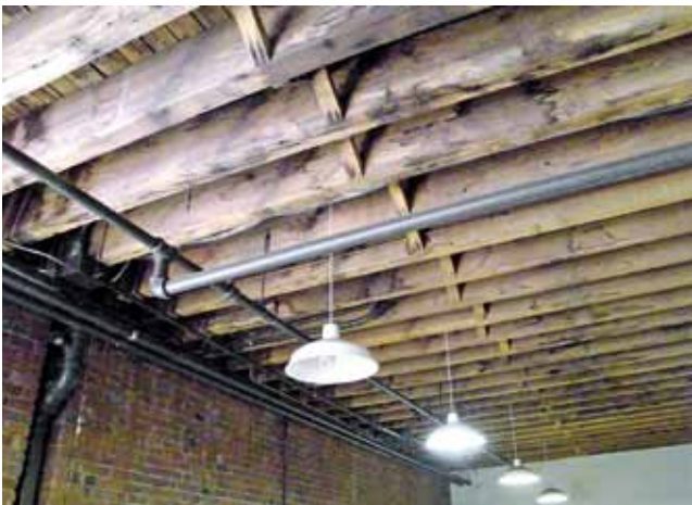
Figure 12: “Ordinary” floors of closely-spaced joists and bridging
