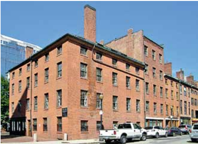
Figure 4: Remains of former warehouses, Central Wharf (now on Milk Street), built 1815–1817
