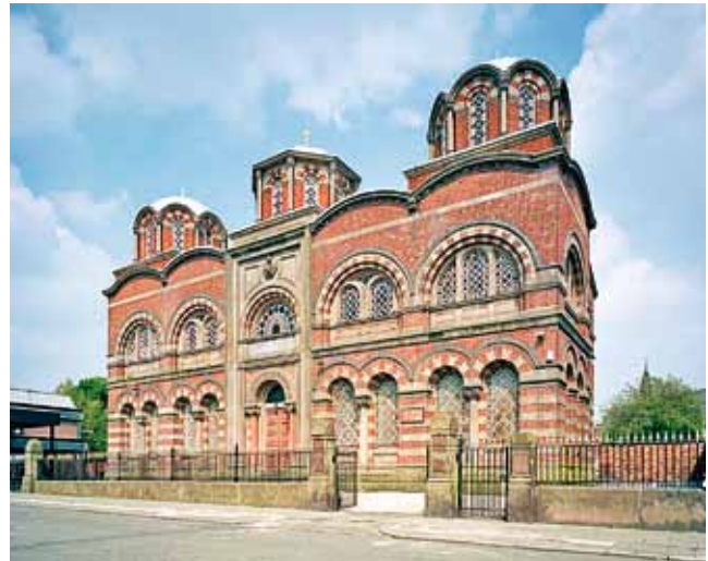
Figure 8: The Greek Orthodox Church in Liverpool (1870)
