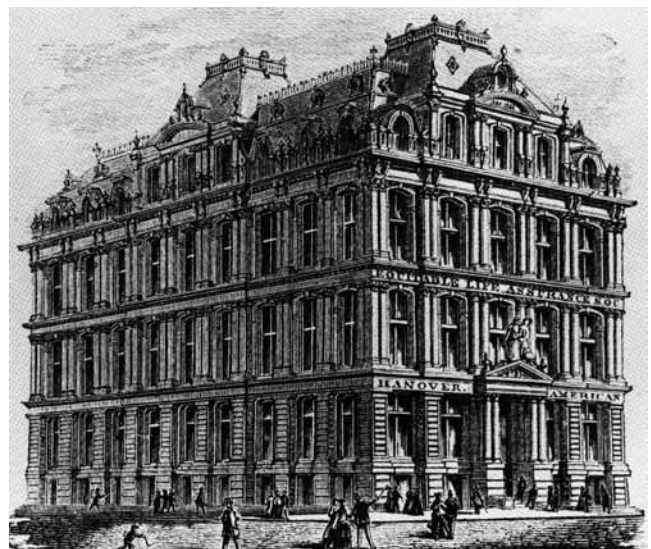
Figure 2: Equitable Building, New York City, by Gilman & Kendall with George B. Post, 1870
