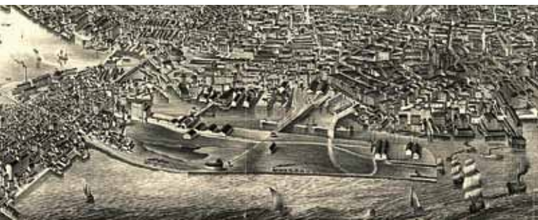
Figure 8: View of Boston Wharf Co. and Commonwealth of Massachusetts's made-land, looking west, ca 1880. The curved piece of land is Fan Pier
