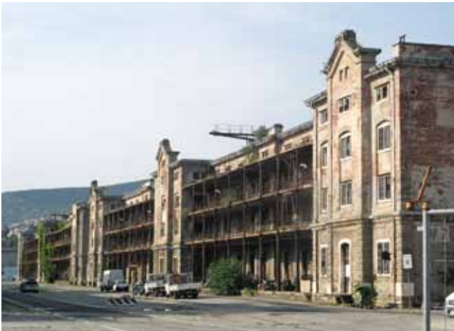
Figure 6: Trieste, Old Port, warehouse no. 7
