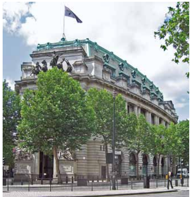
Fig. 18: Australia House, Aldwych, London WC2, A M and A G R Mackenzie, 1913–18
