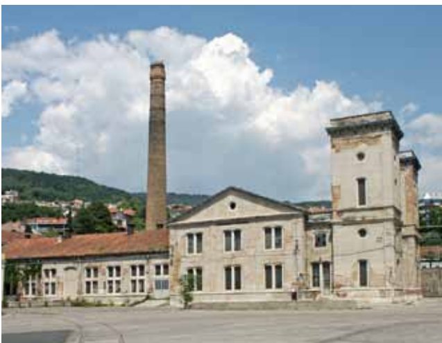
Figure 7: Trieste, Old Port, hydraulic power plant
