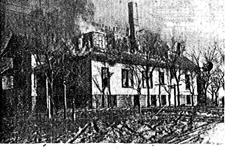
Top story gone, second floor in flames, this is how Hillcrest looked at 5:30. Because they feared the chimney or the roof might fall, firemen kept onlookers at a safe distance and none can be seen in this picture, although a crowd of several hundred were present. Photo by George Jensen.
