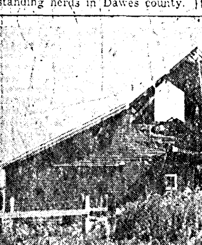
Ed Tvrdek Barn Damaged by Storm
