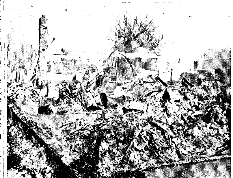
Close-up of the ruins. In the background is the Ord rural fire truck which kept flames from spreading to other buildings. The fire had too good a start to let them do otherwise.—Swopes Photo.
