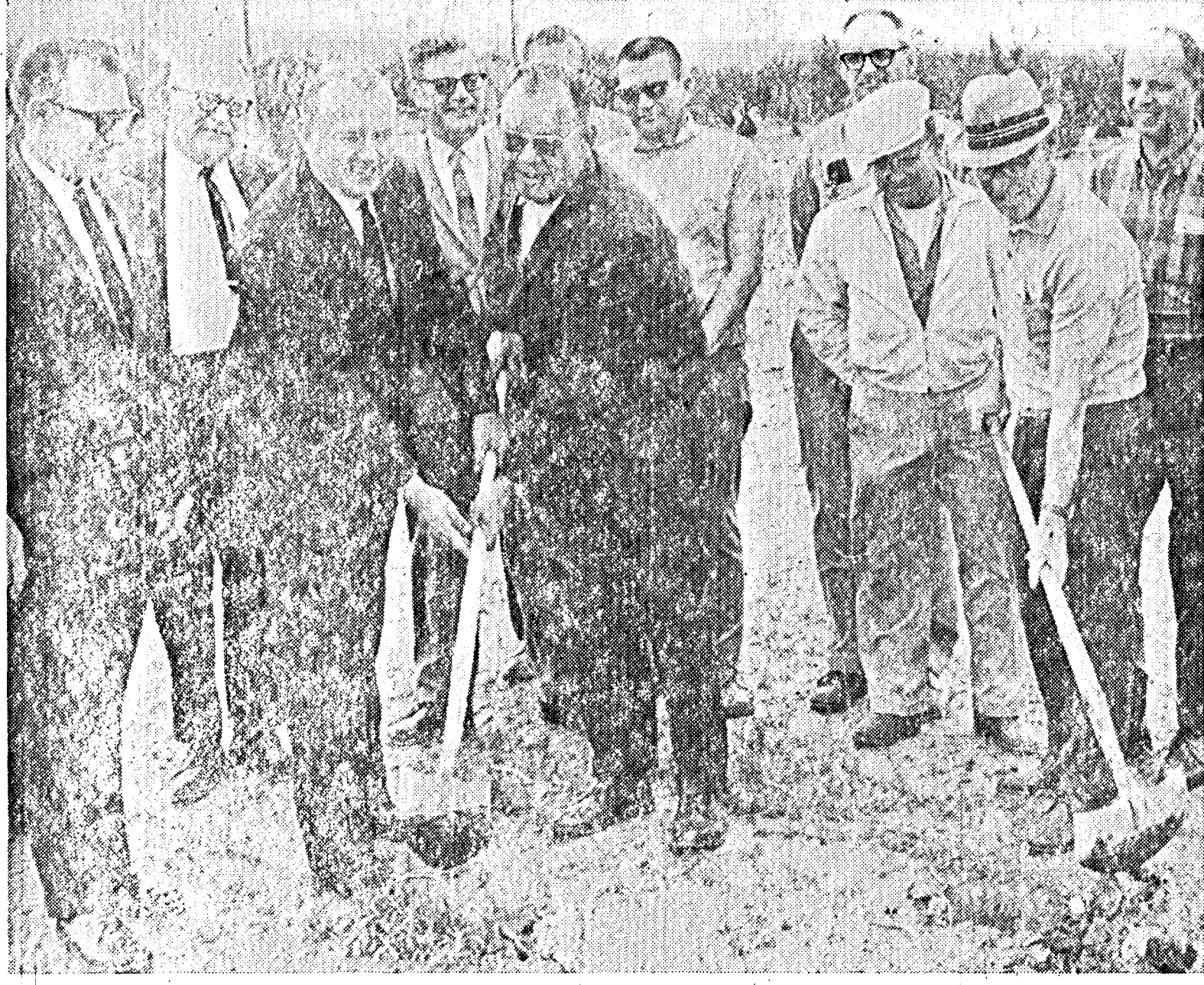
Double shovels bite the dirt to mark the beginning of the new $200,000 Elks Club building north of the golf course. The ground-breaking was held last Wednesday. Construction is expected to be completed in about four months. Manning the shovels were Bill French, chairman of the board of directors, and J. B. Ferguson, exalted ruler of the local chapter, on the left; and Ross Allen, head of the building committee, on the right. Observers included, left to right, Justus Dobesh of Kearney, Howard Huff, Dale Stine, Clayton Calvin, Jack Newland, Henry Janus, Merlyn Van Horn and Cork Greenway. Mr. Dobesh is district deputy grand exalted ruler.
