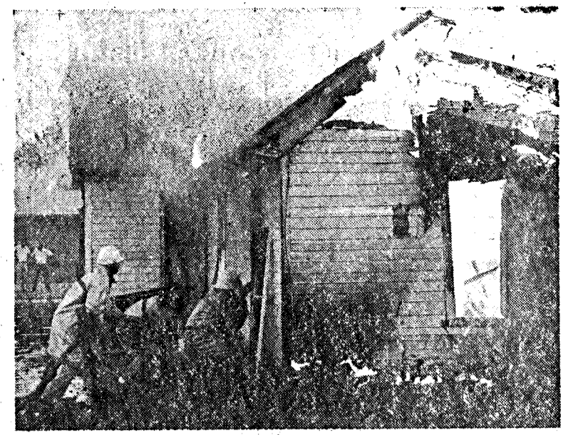
Ord firemen torched the old Grant Marshall residence, 1217 Q, last week for training purposes. The five-room frame building was purchased by Kriewald Construction and donated to Ord firemen. Local fire fighters and those from North Loup, Arcadia, Burwell, and Greeley and representatives from the Nebraska Fire Marshal's Office and the Smeal Fire Equipment participated in the exercise. Under the direction of State Fire Marshal instructors, firemen sharpened their skills and learned new techniques.
