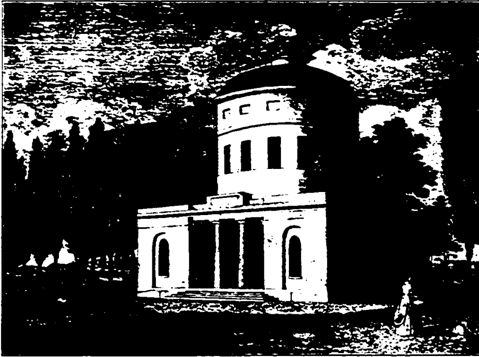
CENTRE SQUARE WATER WORKS
