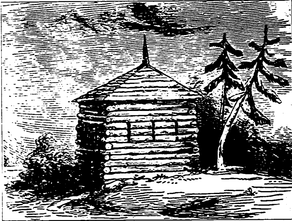
THE BLOCK HOUSE AT WICAGO
