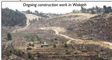
Ongoing construction work in Walajeh
