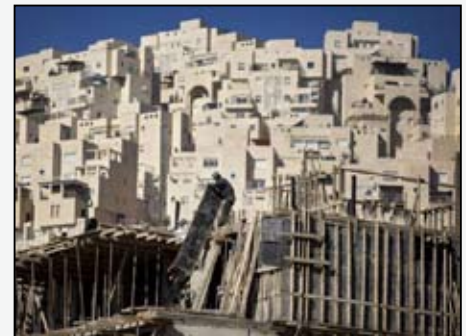
Ongoing construction in Gilo settlement
