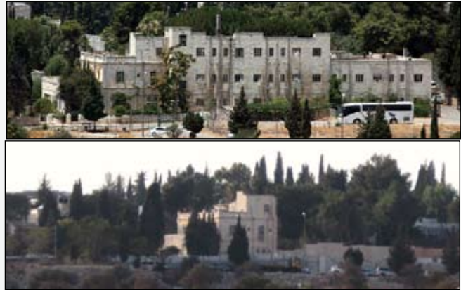
Shepherds Hotel before and after demolition
