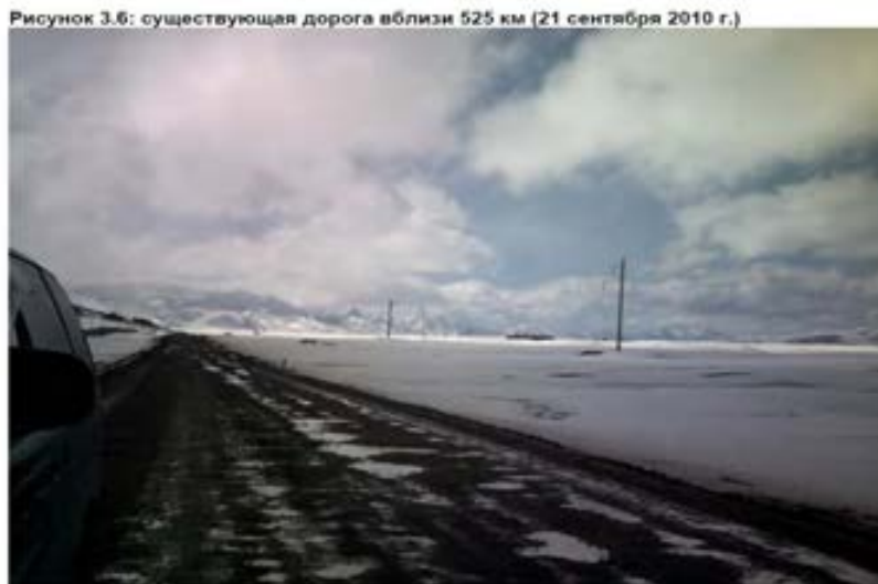
Figure 3.6: Road Condition at KM 525 (on September 21, 2010)
