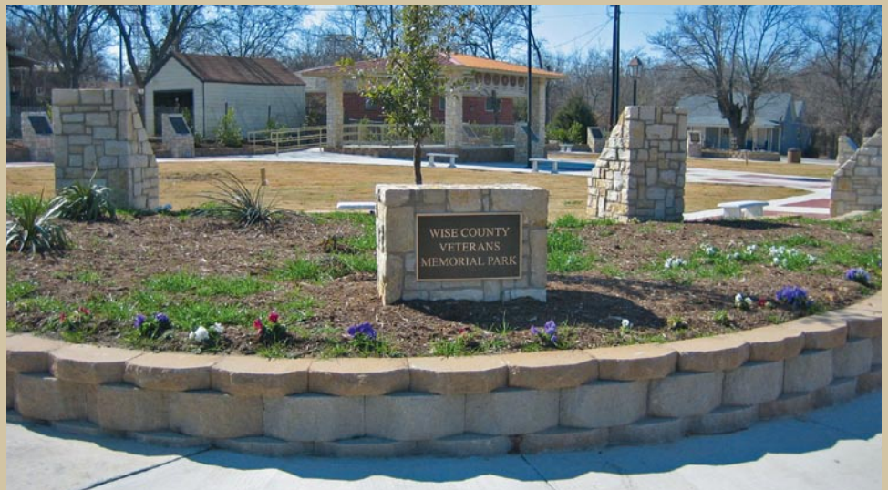
Jewell Concrete’s experimentation with Keystone retaining wall new colors turned out to be a major contribution to the Wise County Veterans’ Memorial.
