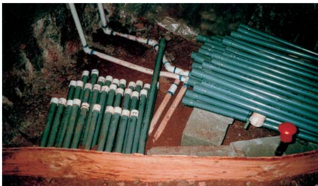
FIGURE 3 A monitoring network should always be installed in a show cave in order to avoid making significant changes in the cave environment. In the case of Kartchner Caverns in Arizona, such monitoring is particularly important because the relative humidity within the cave is close to 100% while outside the climate is very dry. During construction of the pathway, many pipes were laid down and covered by concrete. These pipes contain circuits that connect monitoring sensors within the cave with a computer in the main building. (Photograph courtesy of Arrigo A. Cigna.)
