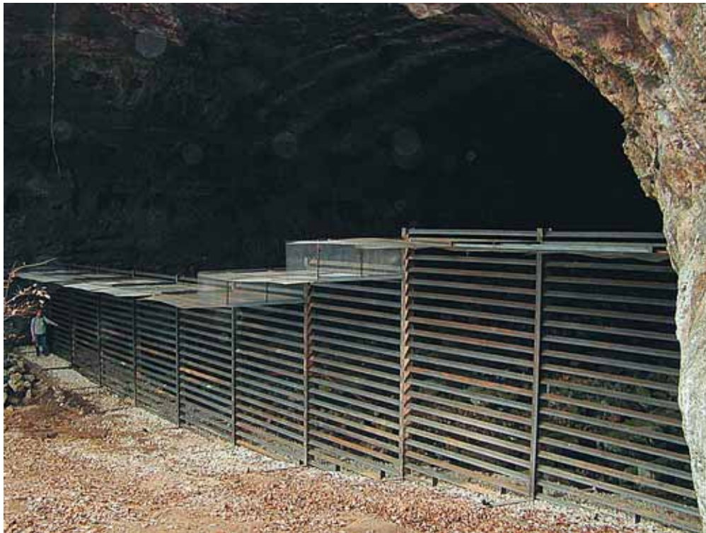
FIGURE 2 The half gate at Great Spirit Cave, Missouri, is 31 m wide and weighs 16 metric tons. It protects gray bats ( Myotis grisescens ) in the summer, Indian bats ( M. sodalis ) in the winter, and many other resources.
