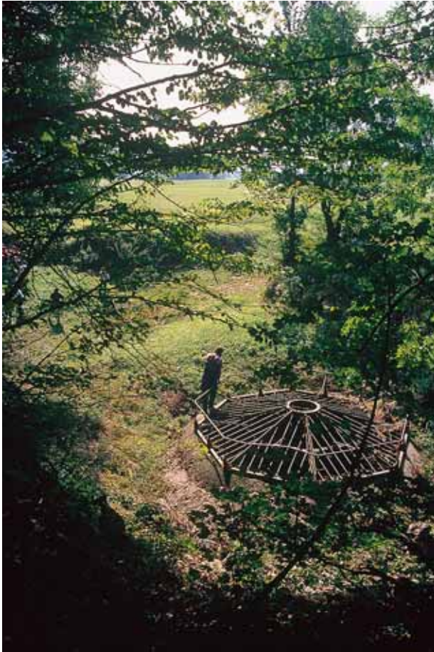
FIGURE 11 A ponor (swallow hole) in the Cernicko polje (Slovenia). The function of the gate is to block coarse debris (in particular, tree trunks and branches) that could impede the discharge of the water.
