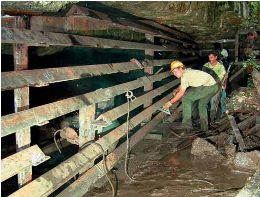
FIGURE 4 A cave-gating class builds a bat-friendly cave gate at McDowell Cave in Missouri. Note the T-bar stiffeners inside the end of the top horizontal bar which provide greater strength and an airfoil design for lower wind resistance. Proper spacing of the bars is essential.
