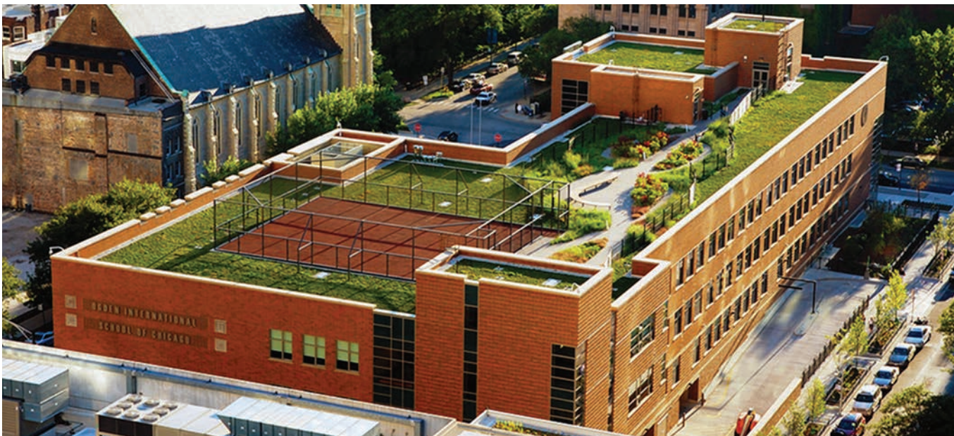
A CCM rooftop garden system on the Ogden International School of Chicago, Chicago, IL.
