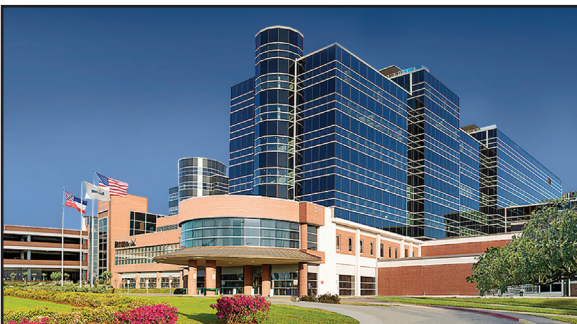
$62M Memorial Hospital Tower Expansion/Renovation ▲ Gulfport, MS
