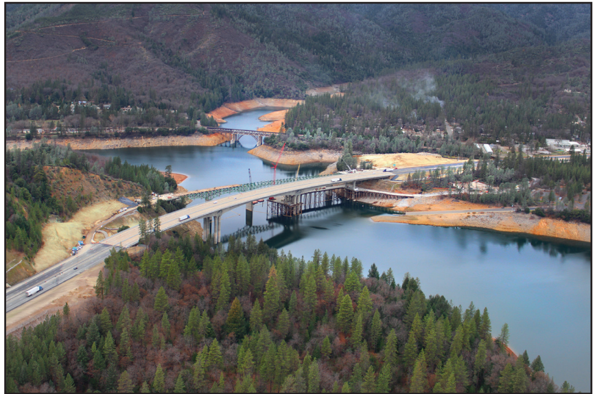
▲ $200M I-5 Antlers Bridge Replacement Caltrans Shasta County, CA
