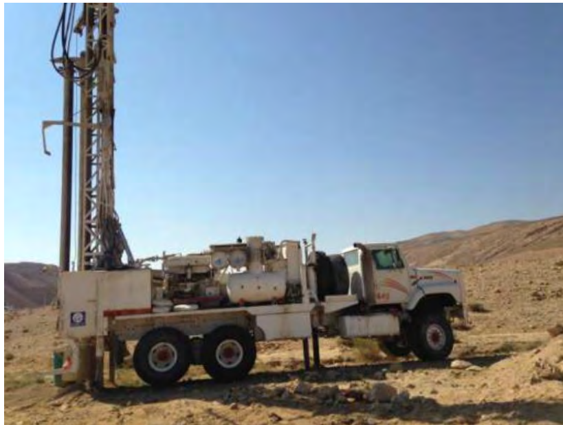
Photo 7.1: Contractor's Mobile Combination RAB/Core Drill Rig
