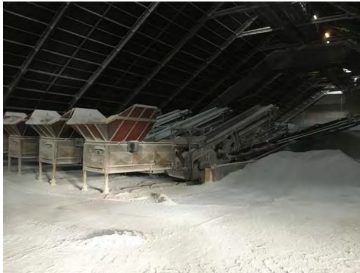
Photo 14.2: Kearton's Building with Mobile Screens and Conveyors at Boulby
