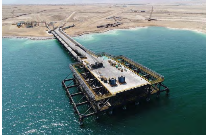
Photo 13.1: DSW Pumping station P9
