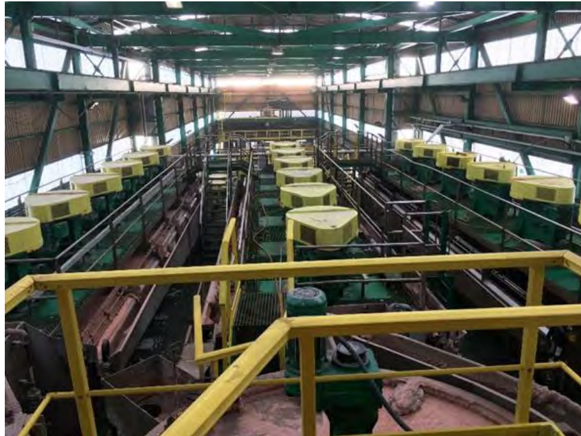
Photo 14.3: Coarse Rougher Cells at the Súría Plant
