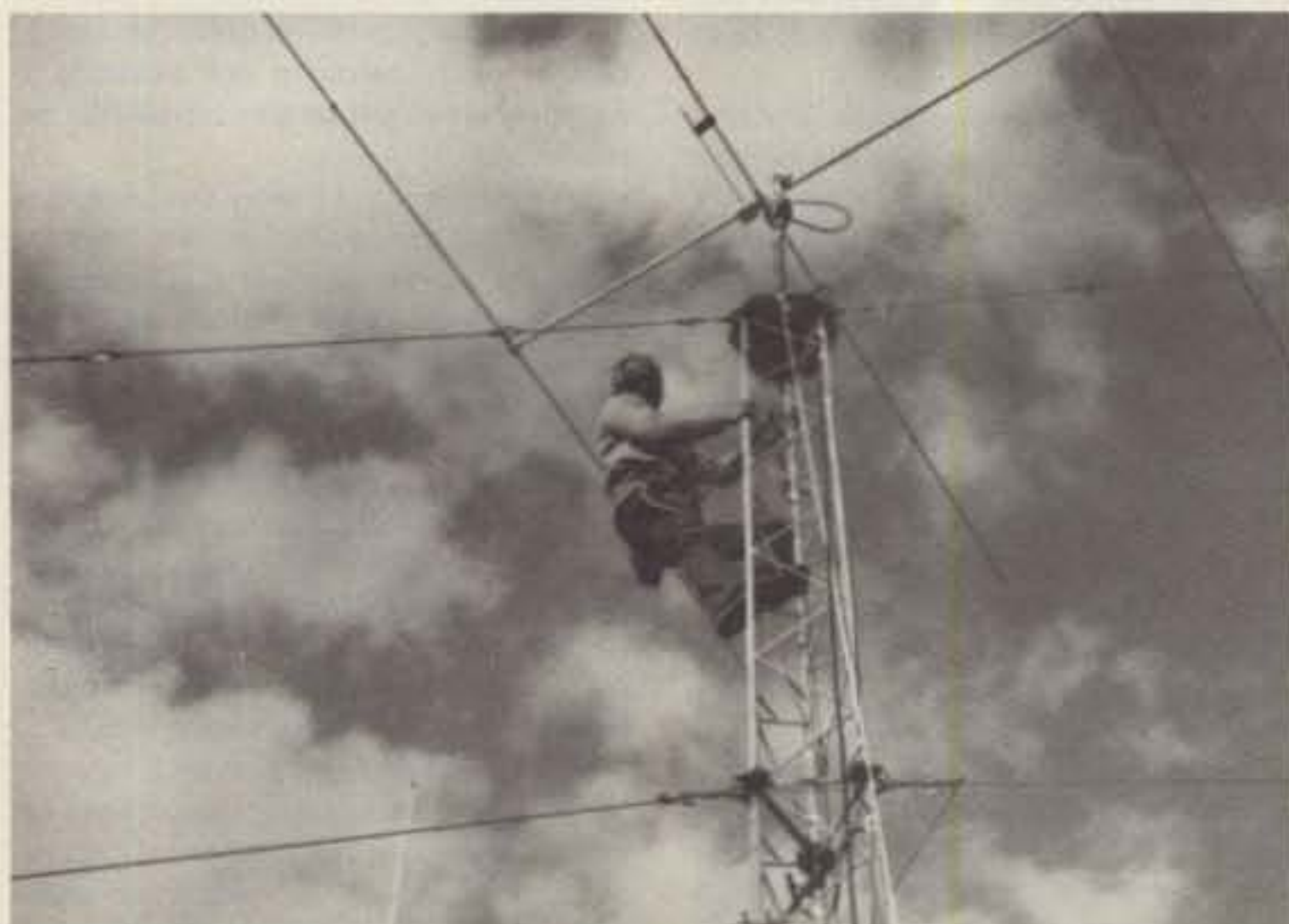
5B4CV doing some antenna work.
